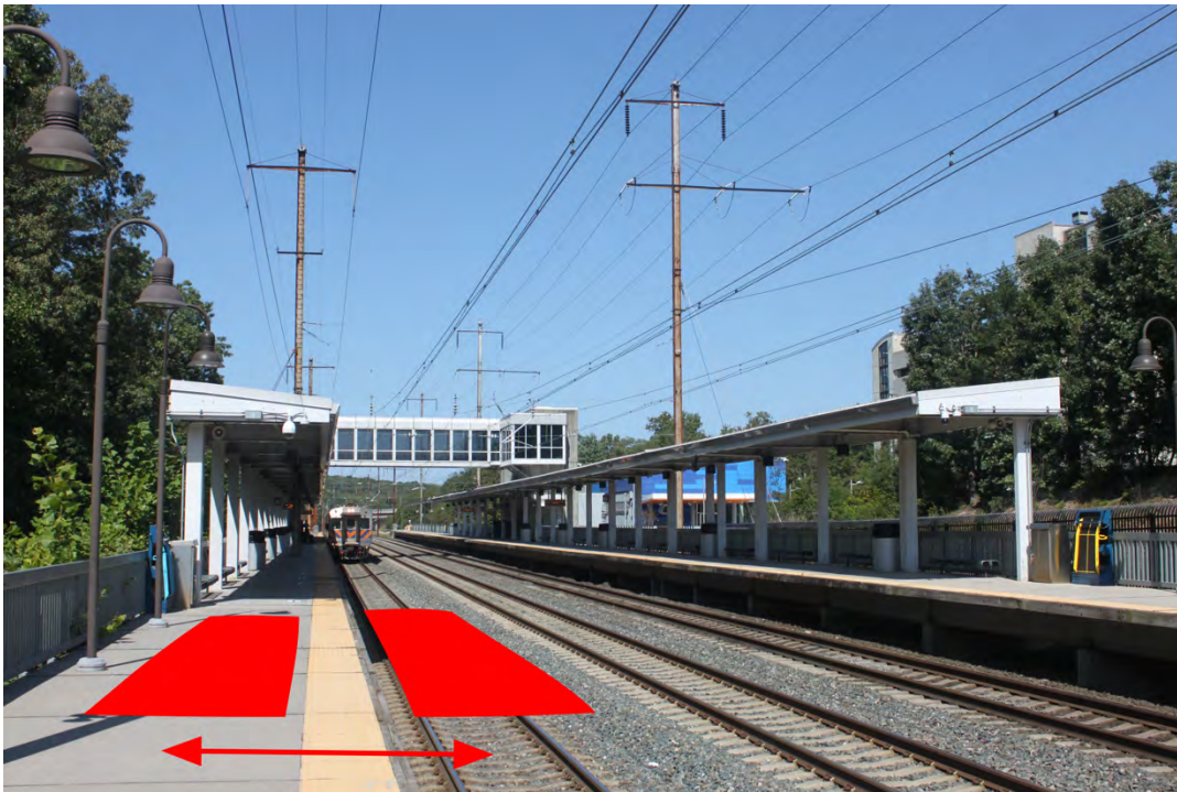
Image 4: BWI Rail Station needed platform reconfiguration
