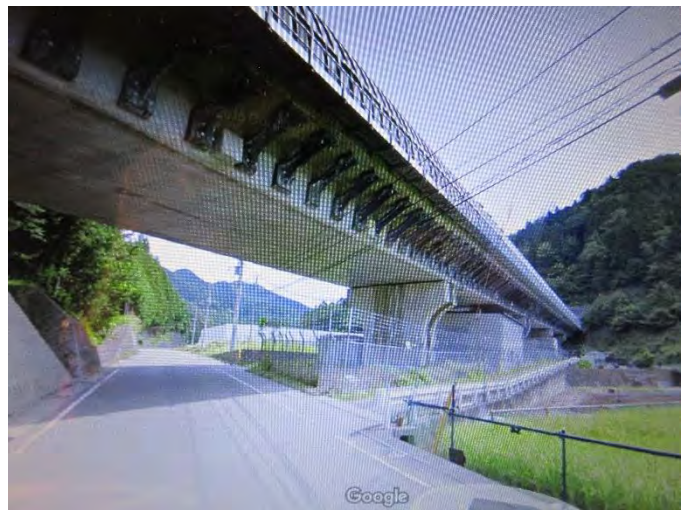
Reality - SCMagLev viaduct fencing in Japan - photo 2.
