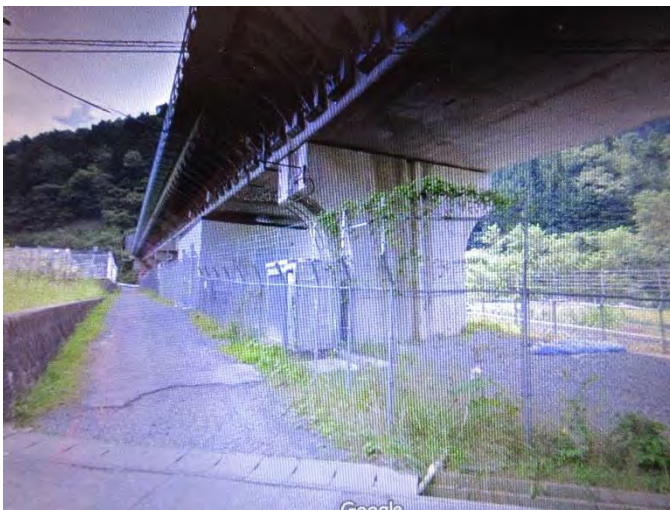
Reality - SCMagLev viaduct fencing in Japan - photo 1.
