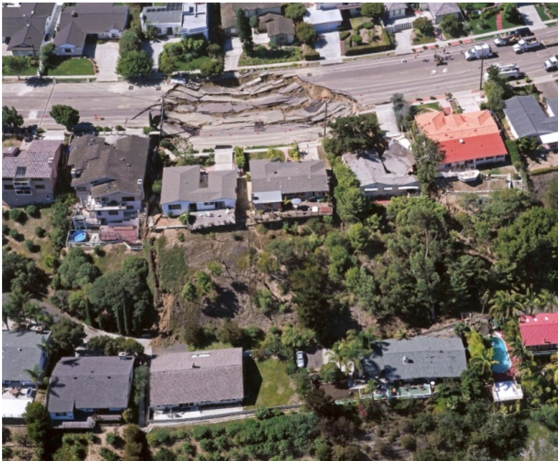
FIG. 2. Aerial View of October 3, 2007 Landslide Photo From Geo-Tech Imagery Intl.
