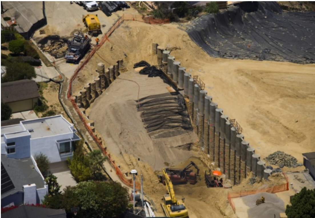
FIG. 7. Roadway Stabilization (Looking North) Photo From Geo-Tech Imagery Intl.
