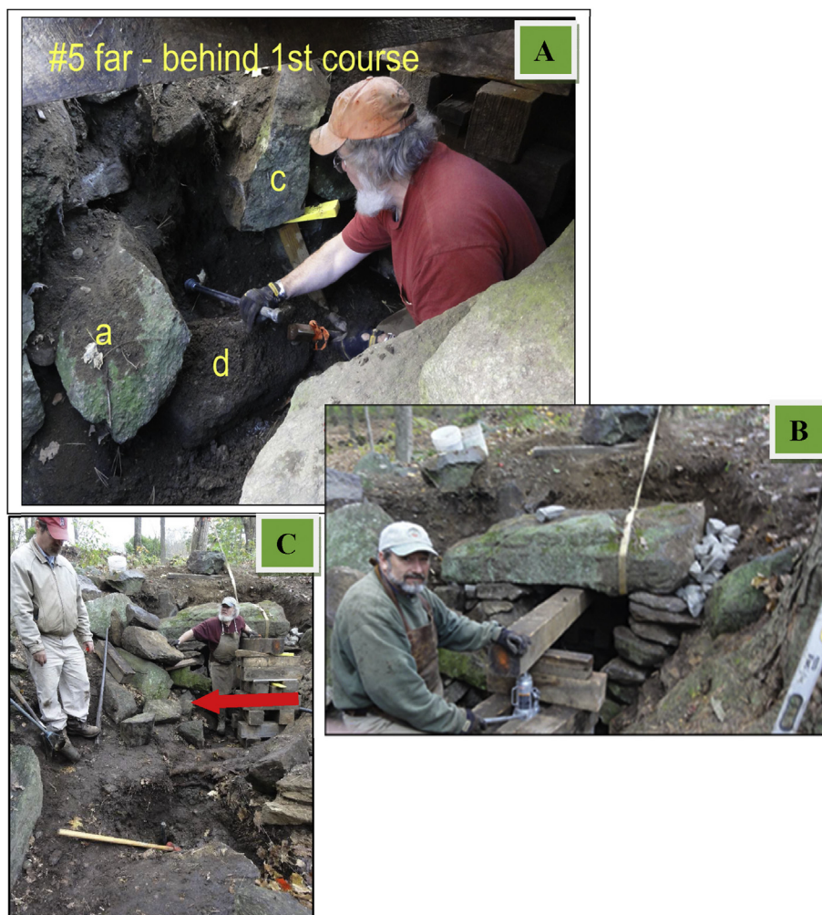
Fig. 3. A. David Stewart-Smith hammers the steel pipe into which sediment for OSL dating will be collected behind stone “d” of the first course in the entranceway to the chamber. B. Peter Wiggin shores up the entranceway to Upton Chamber during repairs. C. Upton #9 and #10 were taken in front of the entranceway with archeologist Marty Dudek (arrow points to OSL collection pipe). All photos provided by Fredrick Martin from Martin (2011b) .
