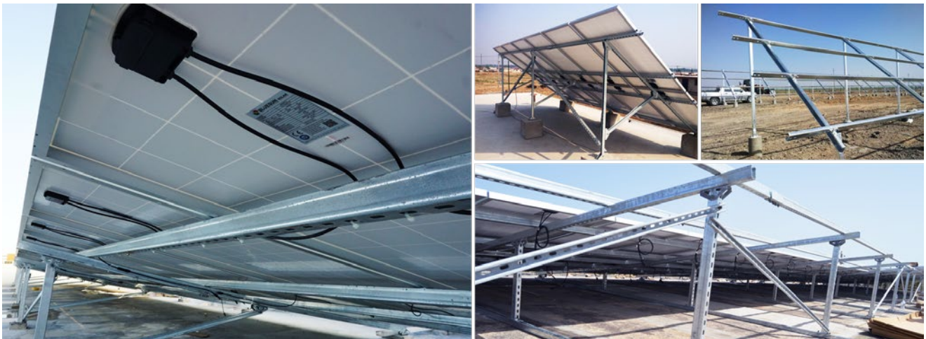
Mounting rail、 Main beam、 Diagonal brace、 back support
