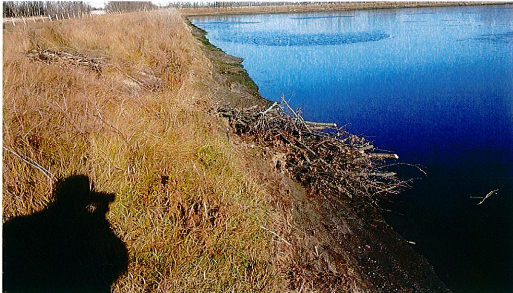
Photo 7 – North berm, inner slope, beaver dam.
