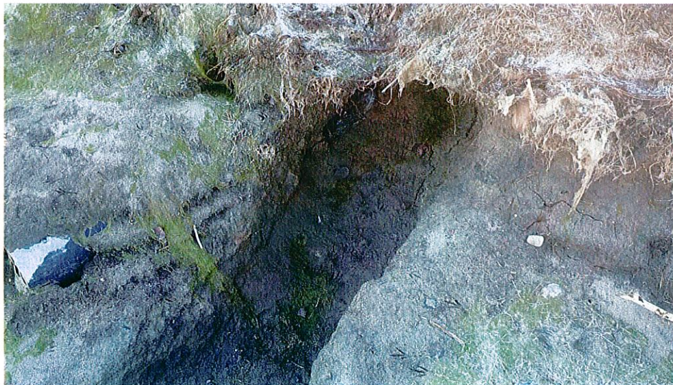
Photo 6 – South berm, inner slope, animal activity borehole.
