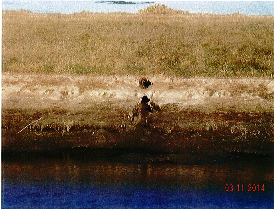
Photo 5 – Central berm, south slope, animal activity borehole.
