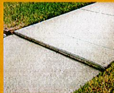
SIDEWALK TRIP HAZARD
