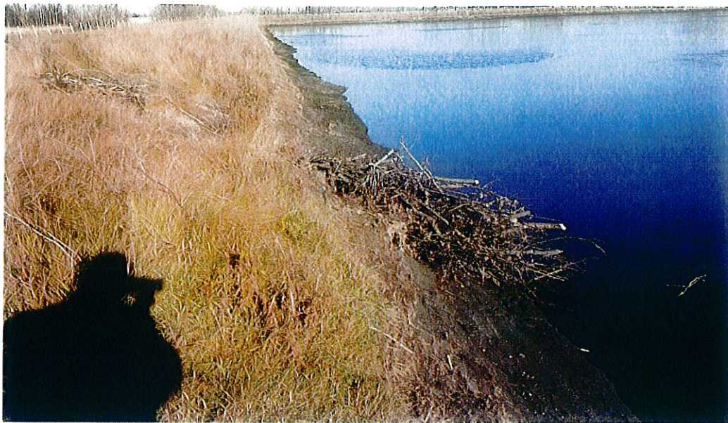
Photo 7 – North berm, inner slope, beaver dam.
