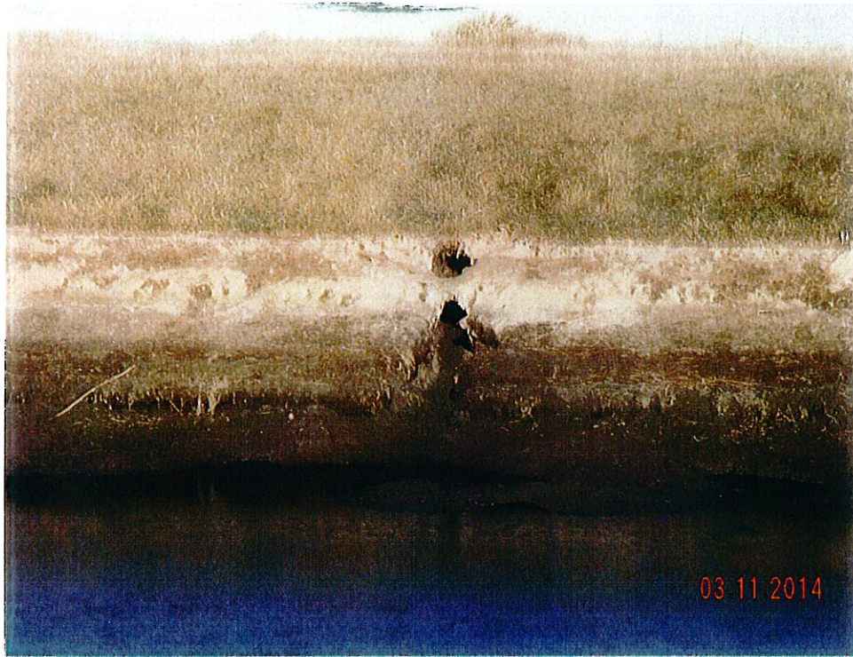
Photo 5 – Central berm, south slope, animal activity borehole.
