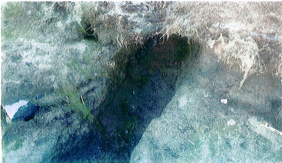
Photo 6 – South berm, inner slope, animal activity borehole.
