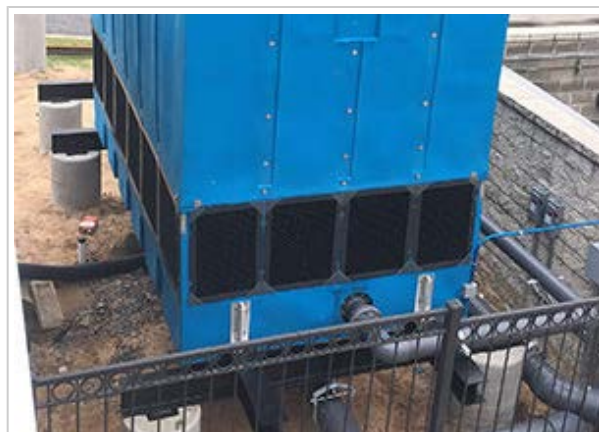
Delta Cooling Towers recently introduced a line of towers constructed of anti-microbial resin.
