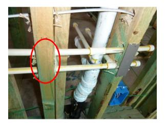
8. We observed a broken brace in the wall at the master suite, where a notch had been cut in the brace for the air conditioning refrigerant lines.
