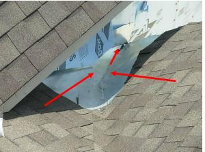
We lifted the edge of the shingles to verify that the tar paper underlayment was properly lapped on top of the drip edge flashing, and it was. No repairs are needed.
