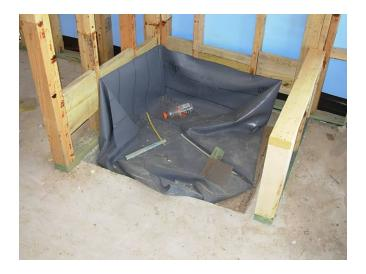
Another typical detail that we see repeatedly on new houses, is a lack of proper and adequate access under the whirlpool tub at the master bathroom for access to the water piping and drain. It is recommended that you check with your builder concerning the tub so that proper access can be built into the tub here at the framing stage of construction.
