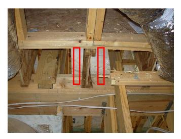
6. We observed that cripple studs were missing above many of the windows and it is recommended that they be installed to provide proper support for the loads above the windows.
