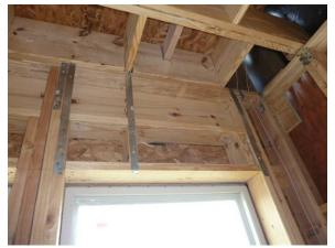
11. We observed major beams in the house which are connected together with bolts. However, many of the nuts were missing from the bolts, and need to be installed.
