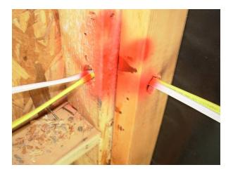
2. We observed in the bedroom between the garage and the master bedroom closet that a diagonal brace has been removed, and some of the studs that were notched out have been replaced. Further investigation with the builder is needed concerning the missing diagonal brace, which is an important framing member, and why it has been removed. (see photos below)
