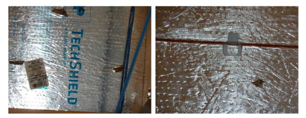
We observed that the nails used to secure the shingles to the roof deck were penetrating the roof deck, and were visible from the attic. This shows that the roofers used nails rather than staples, and that the nails were a proper length.
