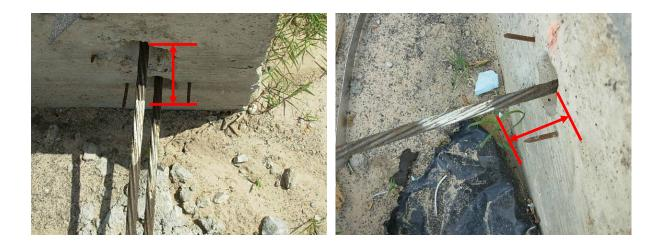
Photos of the anchoring wedges installed in the anchor. The cable ends will be cut off inside the face of the concrete grade beam, and will be covered by grout.
