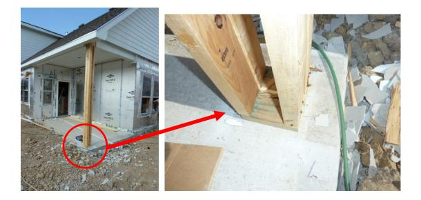
10. We observed wind uplift clips and straps to have been installed at the bottom of the wall framing to attach the wall framing to the foundation; at the top of the wall framing to attach the walls and roof framing; and at windows. The clips and straps were properly installed with no repairs needed.
