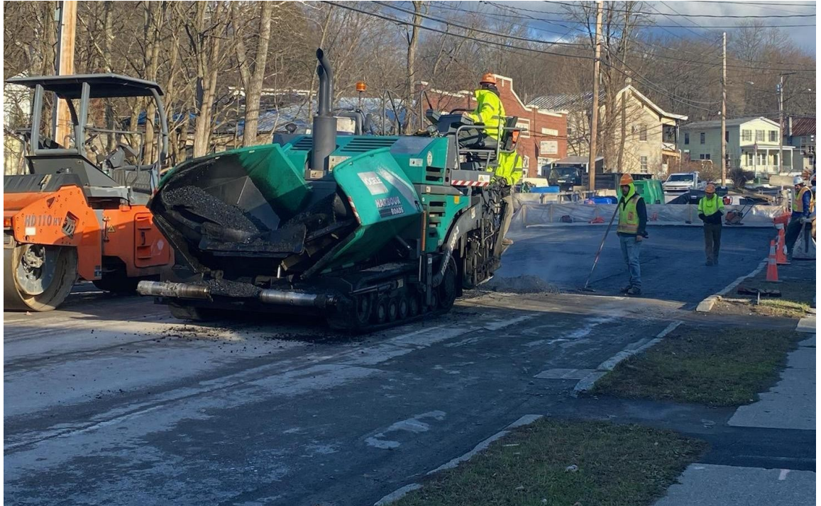
Unforeseen issues have delayed the County Route 23B bridge project in Cairo and ultimately the bridge's reopening.
