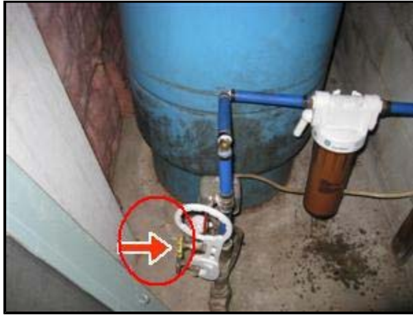
4.3 Picture 1 In basement
