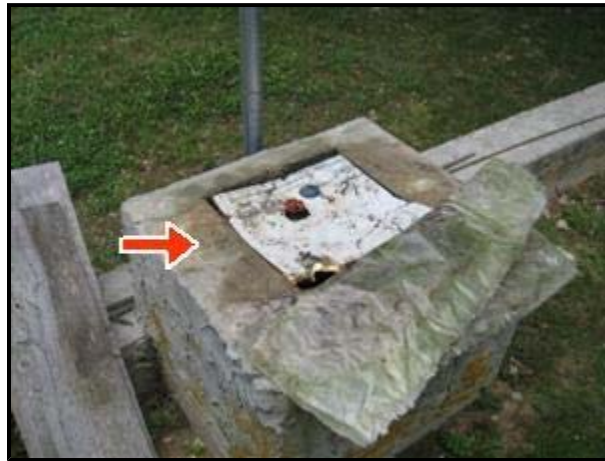
4.1 Picture 3 Well head
