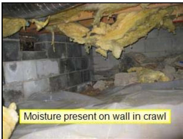
1.0 Picture 5 crawlspace under kitchen
