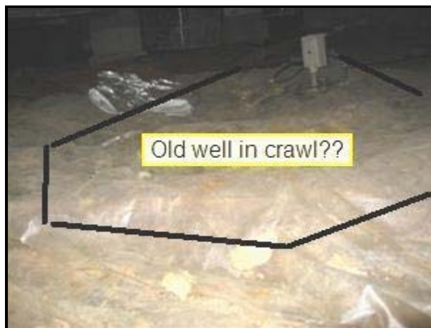
2.6 Picture 2 in crawlspace under new addition
