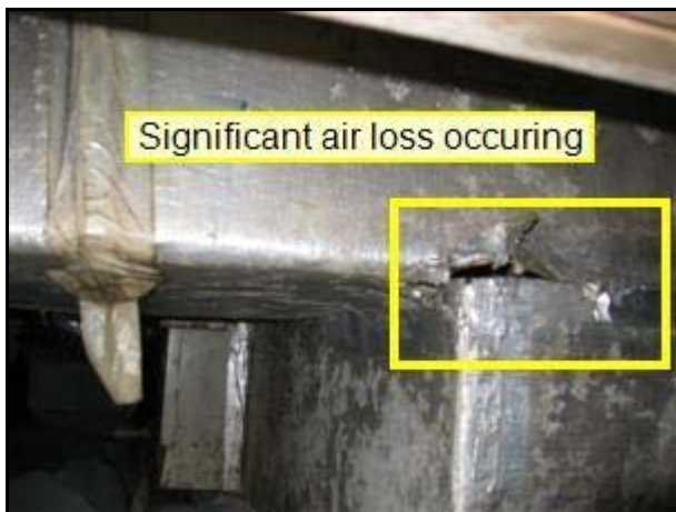
6.3 Picture 4 crawlspace new addition
