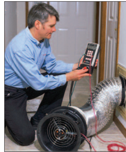
An HVAC inspector can tell you if your ducts are leaking or in need of insulation. Photo by: Julep67Weimer
