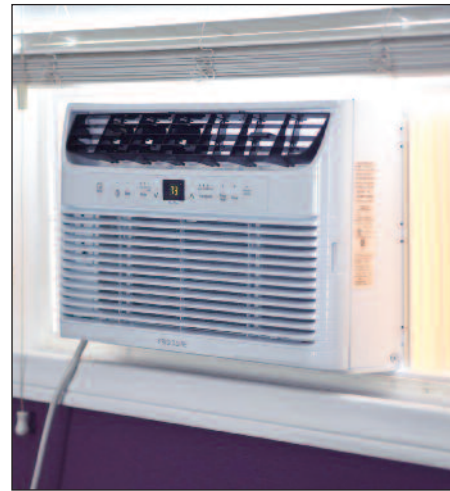
A/C unit is installed flat or according to manufacturer's directions, so that it drains properly. Photo by: Your best digs
