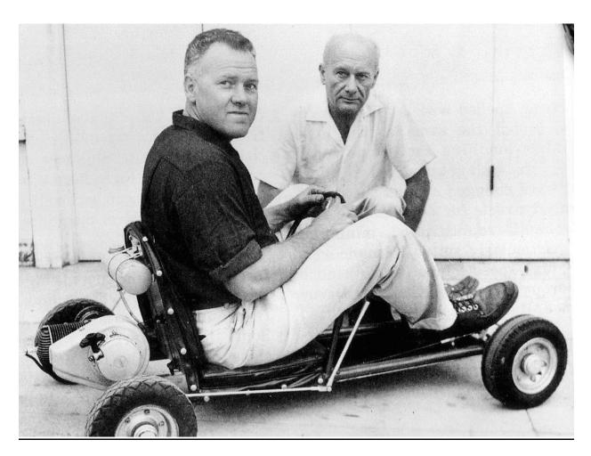
Art Ingels and Lou Borelli with an early prototype of their go kart, which would become known as the Caretta West-Bend (mid 1950s). Early karts utilized small engines designed to be used on chainsaws of the day. (PC: Radne)
