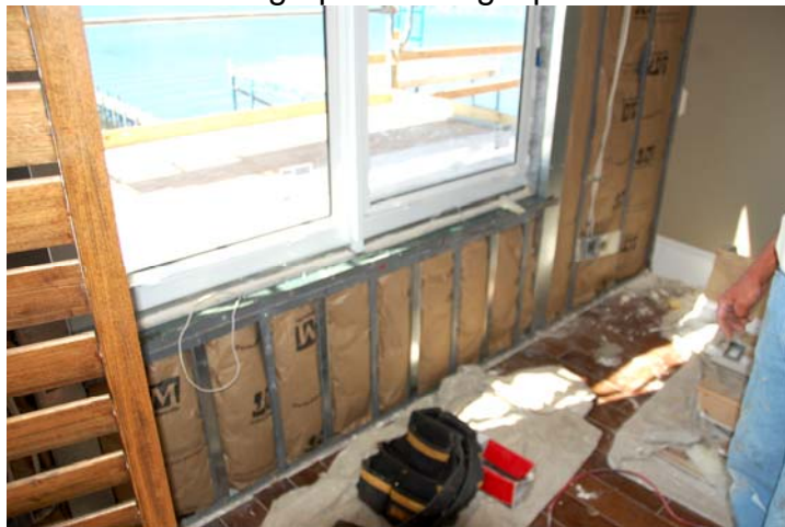
Galvanized metal stud-wall at exterior wall construction.
