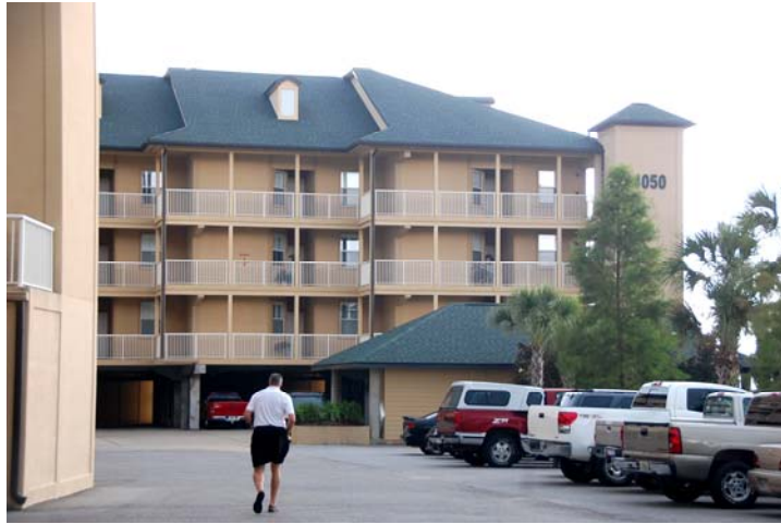
Photograph showing hip roof
