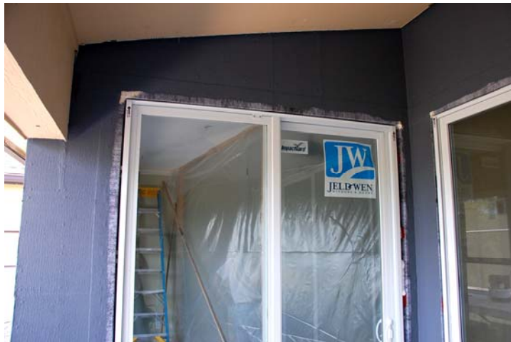
All the windows and sliding glass doors on the end elevations and the waterside elevation were replaced in 2011-12 with large missile resistant glazed products.
