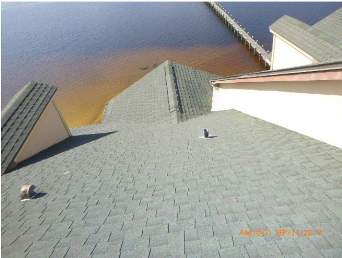
#2 - Predominate Roof Covering - Meets 2001 FBC
