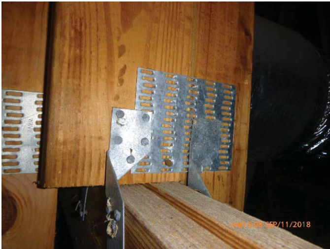
#4 - Roof to Wall Attachment - Hurricane Clips
