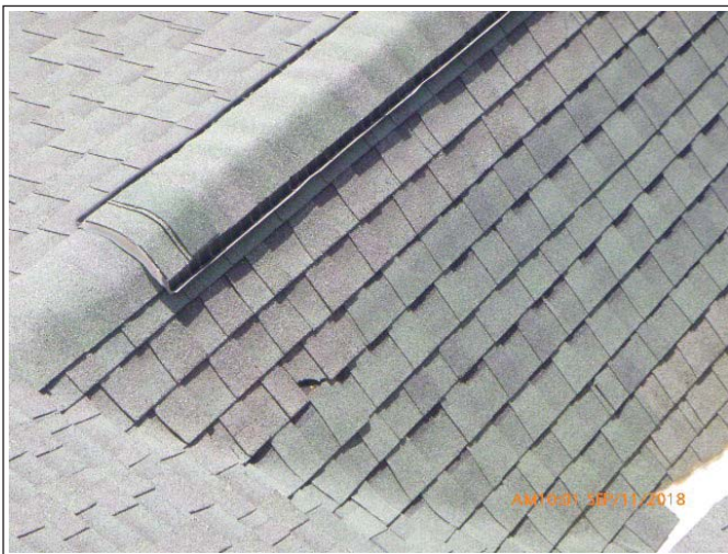
Damaged Shingles
