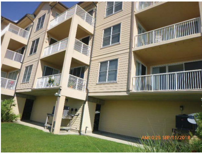
#7 - Opening Protection - None
