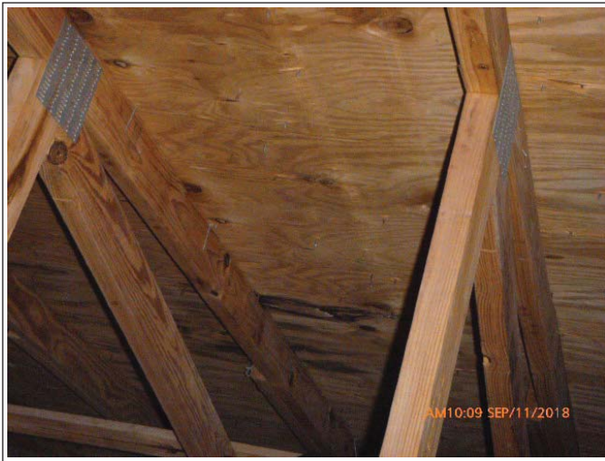
Roof-Leak
