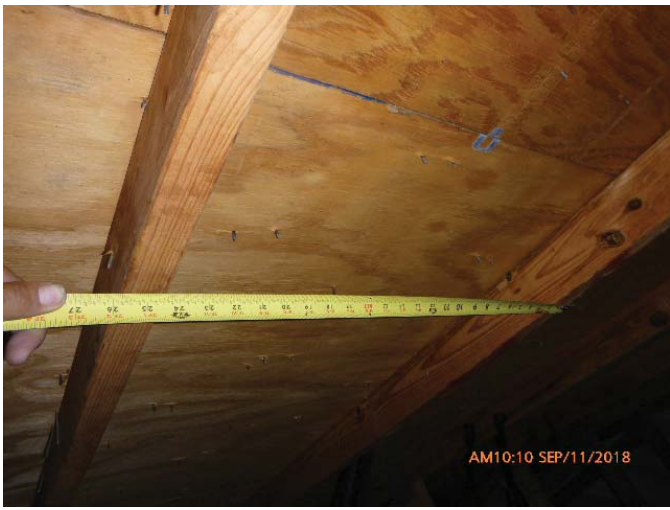
#3 - RDA - Rafter Spacing 24" or Less
