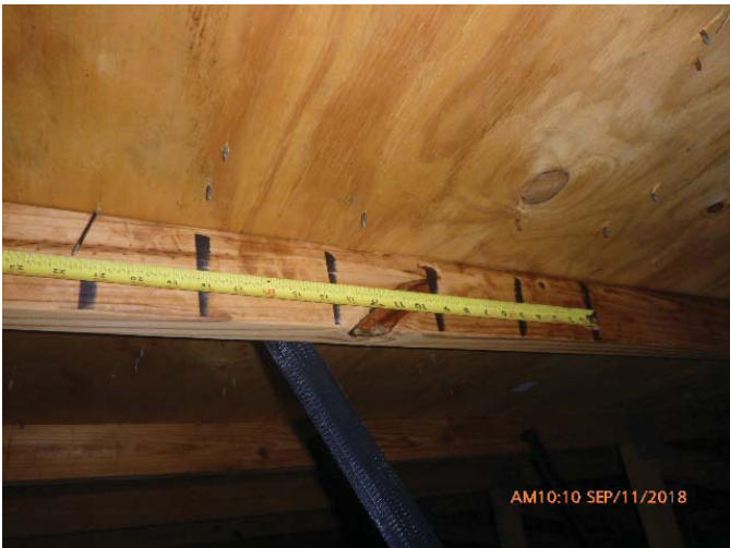
#3 - RDA - 6" or Less Nail Spacing in Field
