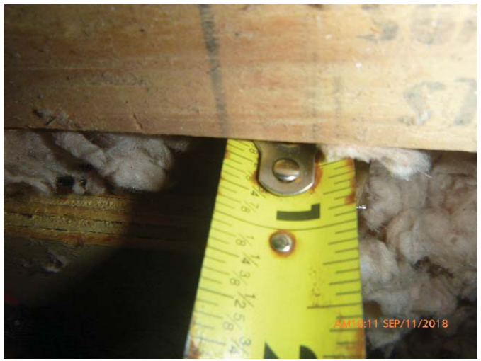
#3 - RDA - Sheathing Thickness 7/16" or Greater
