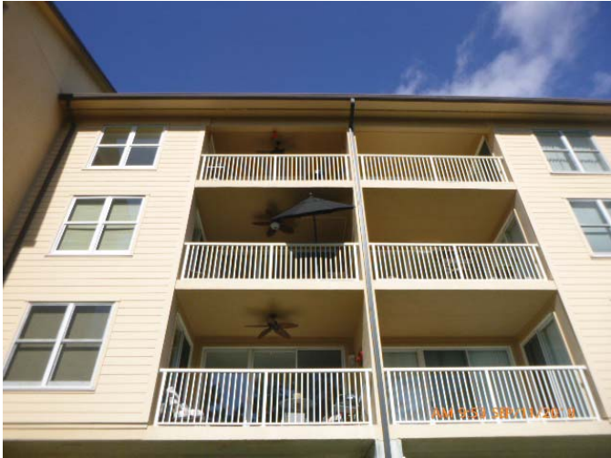
#7 - Opening Protection - None
