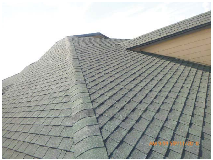
#2 - Predominate Roof Covering - Meets 2001 FBC
