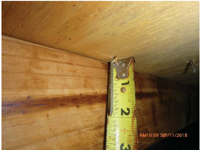
#3 - Roof Deck Attachment - 8d Nail
