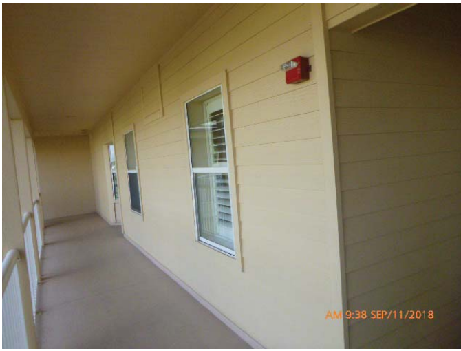
#7 - Opening Protection - None
