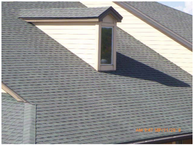
#7 - Opening Protection - None
