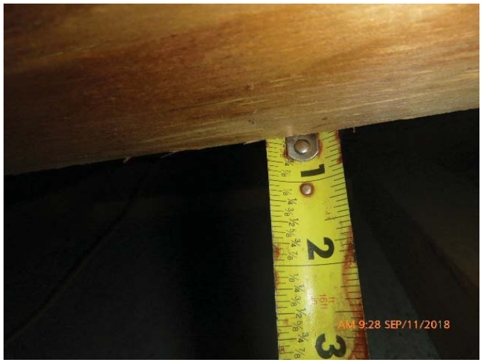
#3 - RDA - Sheathing Thickness 7/16" or Greater
