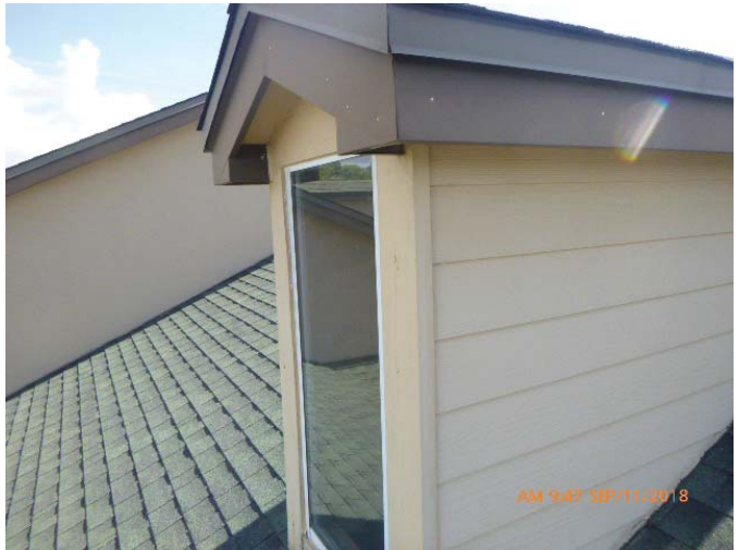
#7 - Opening Protection - None
