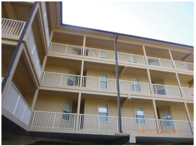
#7 - Opening Protection - None
