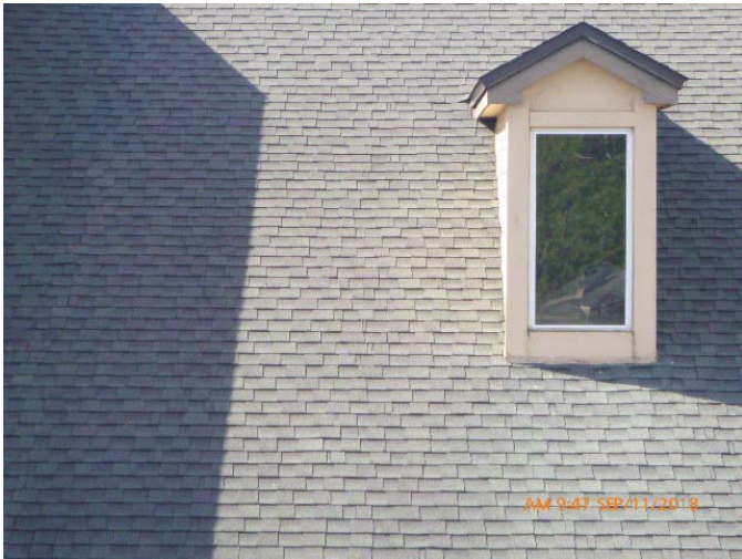
#7 - Opening Protection - None
