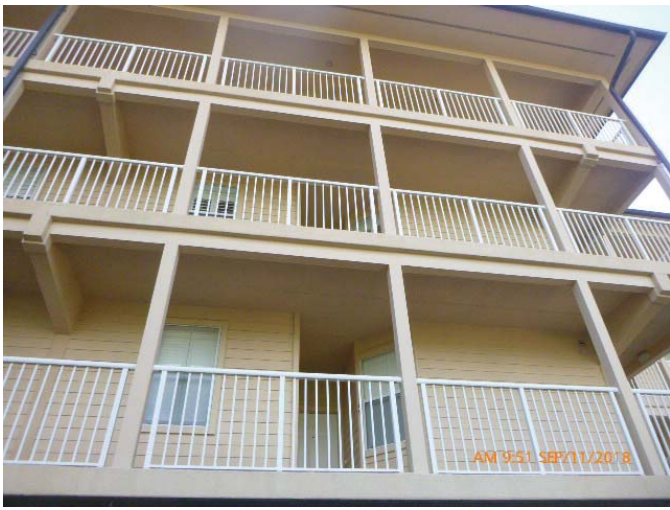
#7 - Opening Protection - None
