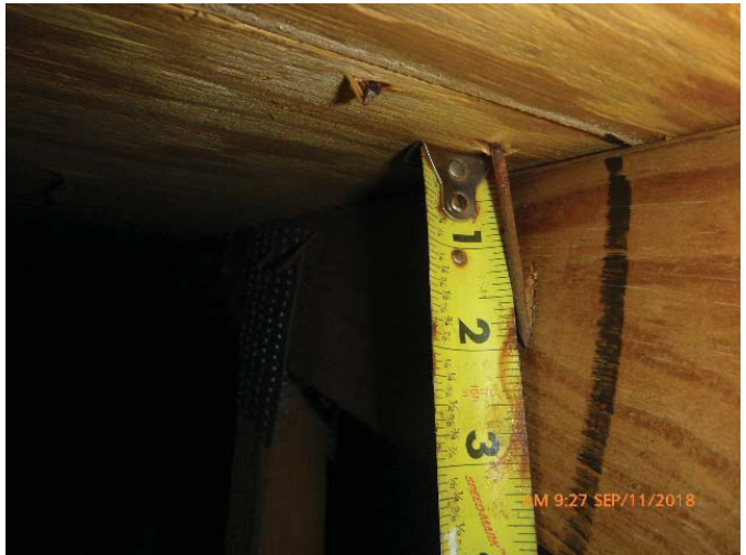
#3 - Roof Deck Attachment - 8d Nail
