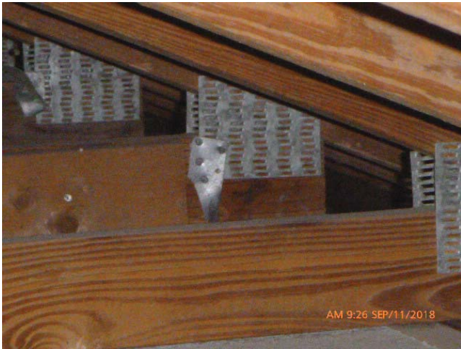
#4 - Roof to Wall Attachment - Hurricane Clips
