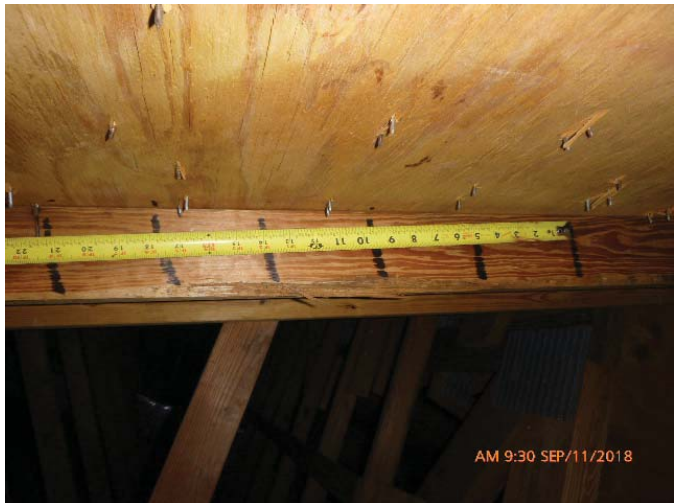
#3 - RDA - 6" or Less Nail Spacing in the Field
