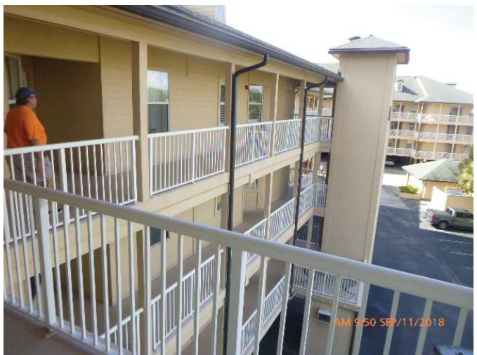
#7 - Opening Protection - None
