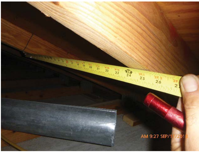
#3 - RDA - Rafter Spacing 24" or Less
