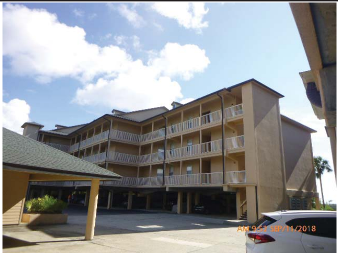
Front & Right of Home
