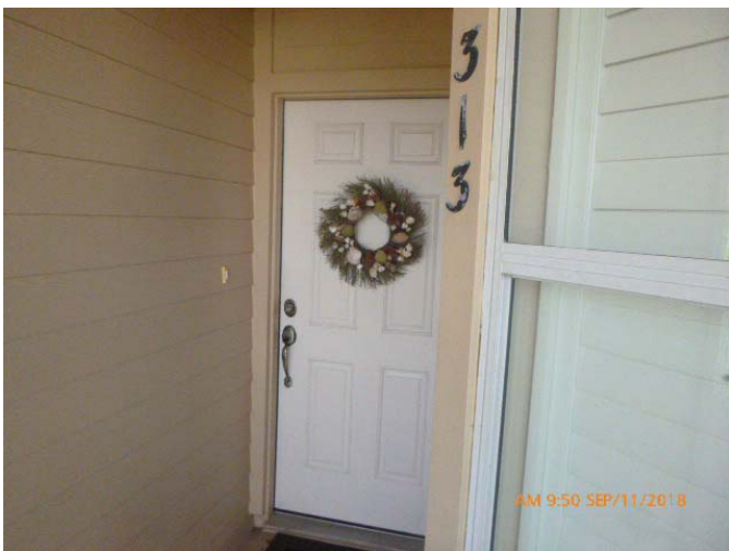
#7 - Opening Protection - None
