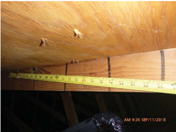
#3 - RDA - 6" or Less Nail Spacing in Field
