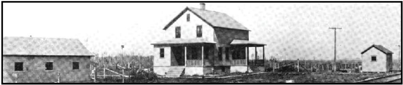
Typical Section Foreman's House with Tool House at Right and Bunk House at Left
