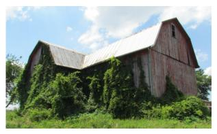
The Present and the Future: The main floor failed along one corner of the barn, causing one side to collapse into the basement. Due to this collapse and weather taking its toll, the Dorr barn needed to be dismantled. Much of the red siding has gone to side the interior walls of a modern day barn. Beams, doors, and boards await future projects.
