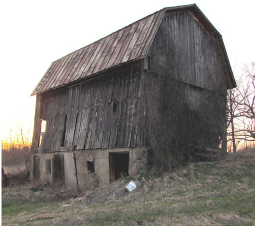
Bulging barn walls
