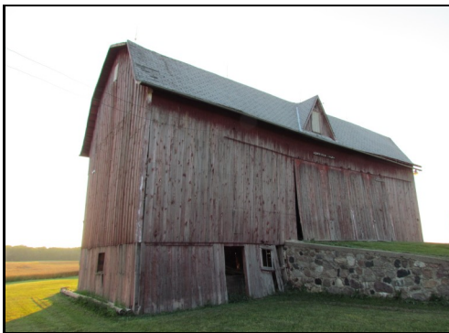
View of embankment leading into the barn,.
