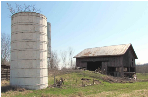
View of embankment on which barn was built.
