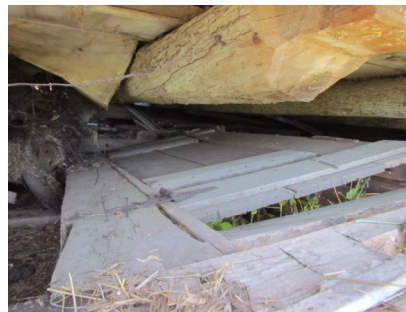
Door beneath the collapsed main floor.
