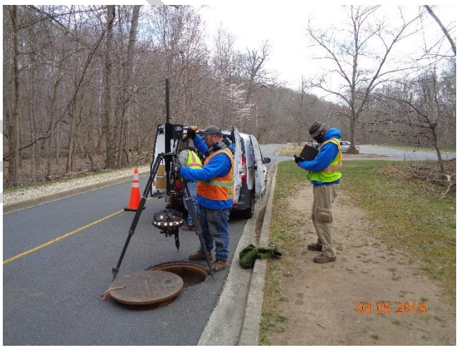
Contractor Deploying Digital Panoramic Inspection Equipment
