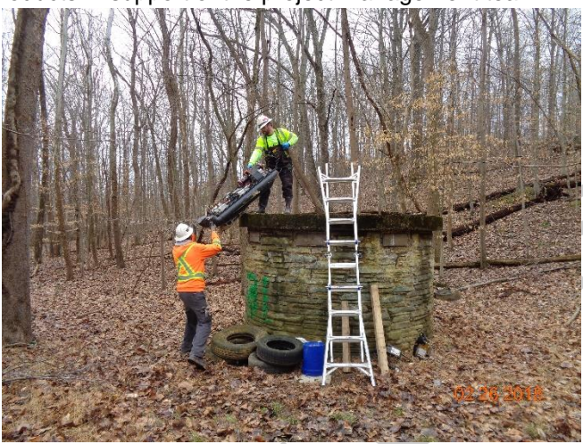
Contractor Deploying Sonar/Video/Laser Inspection Equipment
