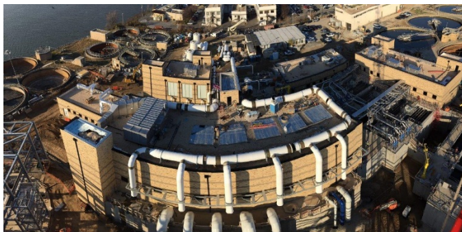
The top image shows the major components of the project. The bottom picture is the pump shaft.
