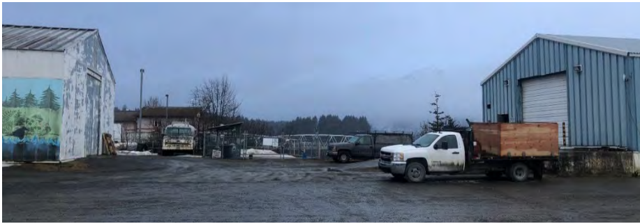
Seldovia Fuel and Lube Building (left), City Office Building (right)
