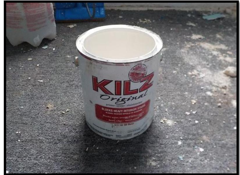
Provide documentation of the type sealer used. (Wood/Drywall=KILZ, Zinsser, Masonry= Drylok)
