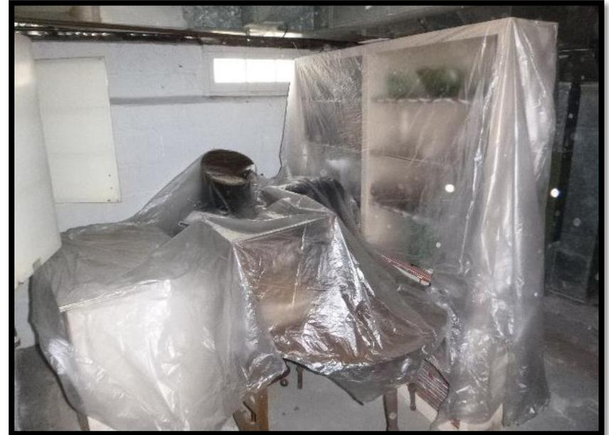
When a room is determined to have discoloration, the expectation is to move personal property into the center of the room so a preservation contractor is able to walk around the room perimeter and spray/treat the walls and ceiling with antimicrobial solution. Thin painters plastic is to be used to cover and protect the personal property from any overspray during the remediation.
