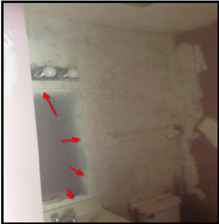
Vendor used spray cans and unprofessionally sprayed across edges of mirror without protecting.
