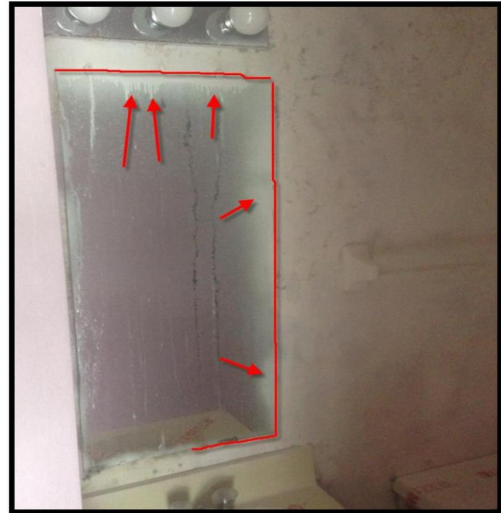
Close up photo showing paint runs on the bathroom mirror. Notice the poor and uneven and thin coverage of the sealed surfaces.
