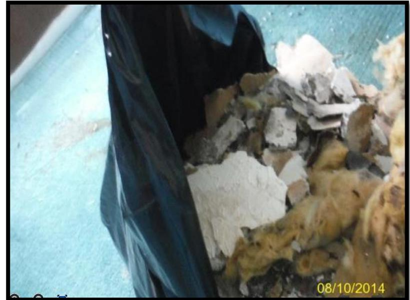
**Debris is properly disposed of by containment in contractor grade bag.**
