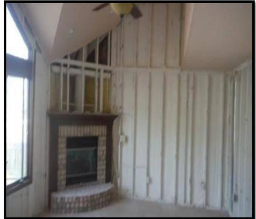
**Vendor did a nice job of sealing the wall cavity discoloration but only applied one coat without prior bleaching.**
