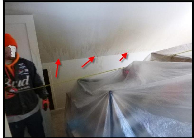
Arrows point to clear lines where the discoloration has begun to appear. This is early stage low density discoloration treatable with “Treat and Seal”. A painter’s drop cloth is to be used to protect carpet when sealing with appropriate primer.
