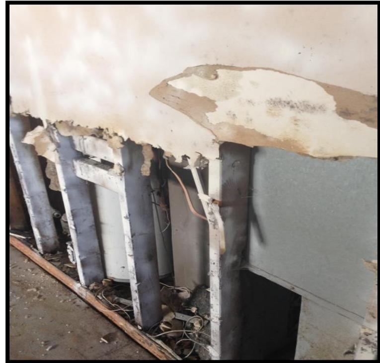
**Wall board is to be cut with a saw or removed at a factory seam to perform a professional demolition service so no additional demolition is required by the renovation contractor.**
