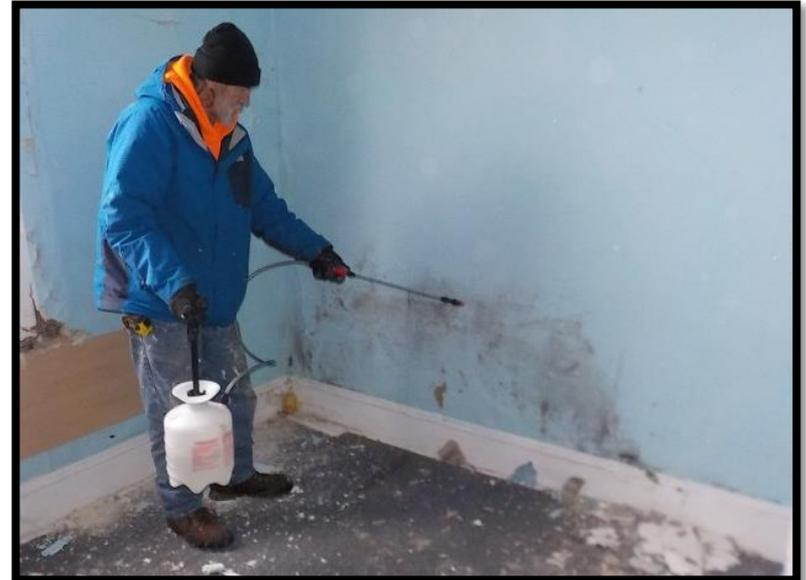
Spray with antimicrobial solution after documenting with photographs: while still on site completing the *Debris Removals* and *Move Personal Property* work items or after a grass cut. Install a label in each treated room when finished.
