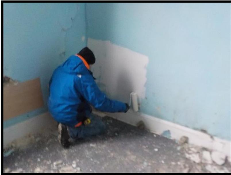
Application of sealer is to be performed on dry wall board after the spore kill has been address through previous antimicrobial spraying. Brush or roll sealer, DO NOT use aerosol spray cans.
