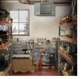
PTP unit heaters can use natural or propane gas, and are available in single-stage or optional two-stage controls.
