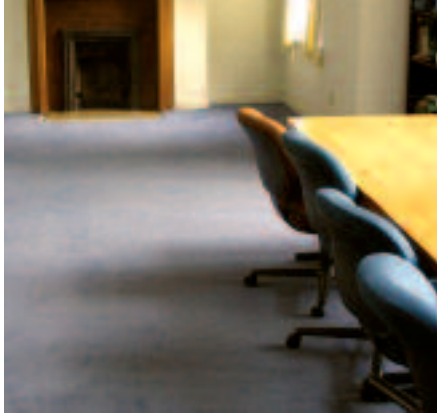
Carpet made from recycled plastic (PET) soda bottles was installed in the EarthWays Home.
