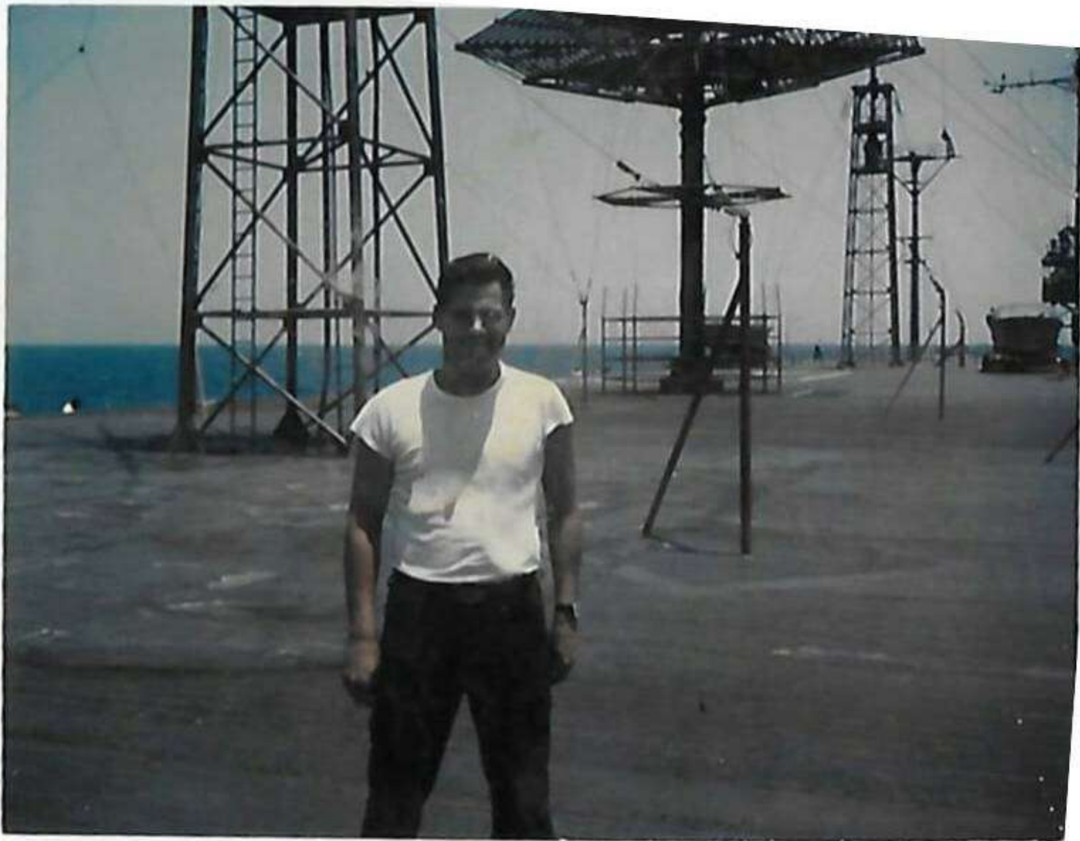
Me on the Antenna Deck.
