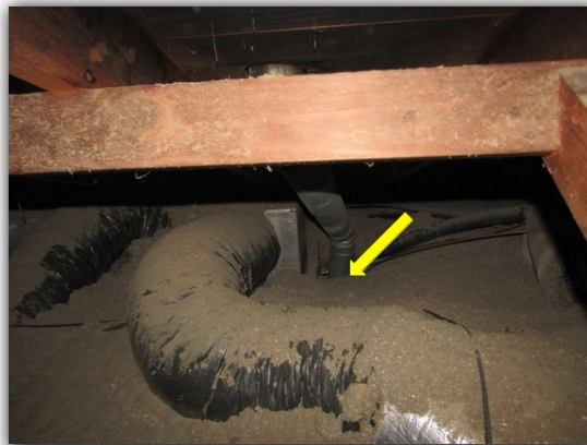
Flues for furnaces contact insulation
