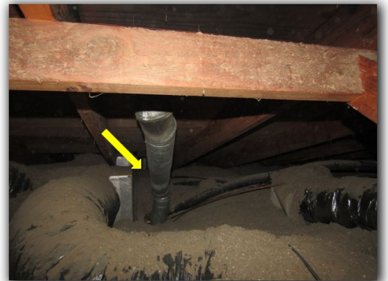
Flues for furnaces contact insulation
