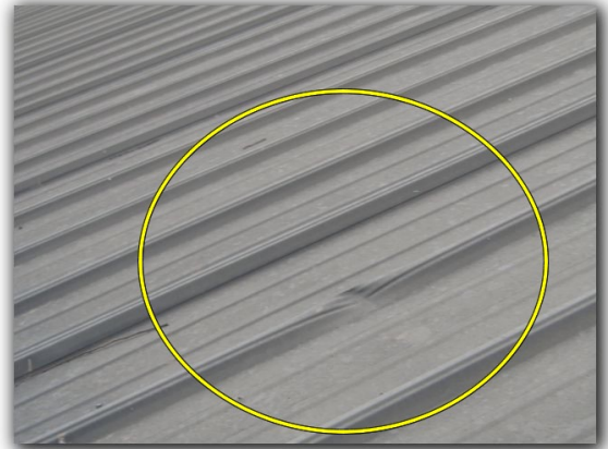
Multiple dents in roof observed
