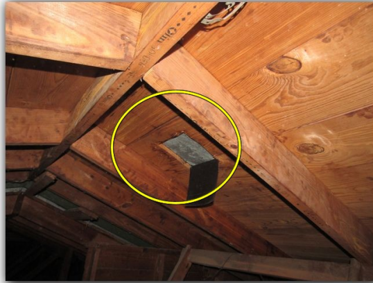
Evidence of past leaks observed in attic
