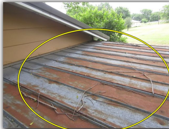
Rust observed on roofs for back and side porches
