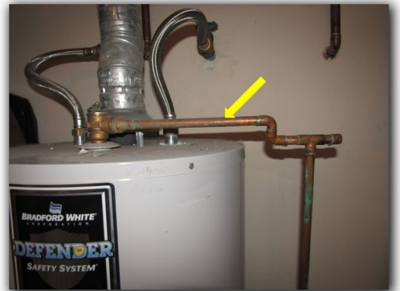
TPR drain line for hall bathroom water heater appears to be too small
