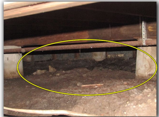
Possible poor drainage in crawlspace. Appears water may enter crawlspace and pool in multiple locations in crawlspace.
