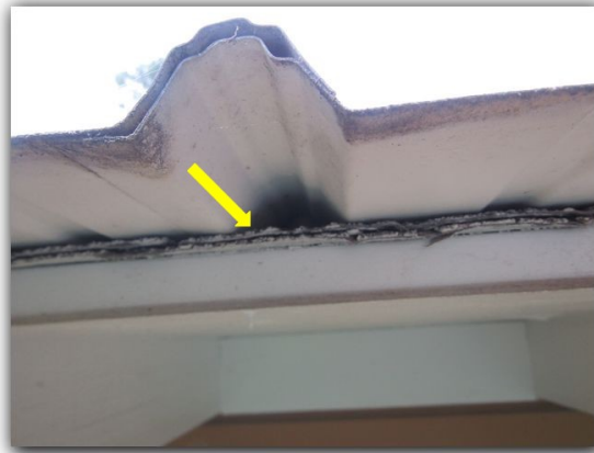
Appears metal roof is installed over asphalt shingles
