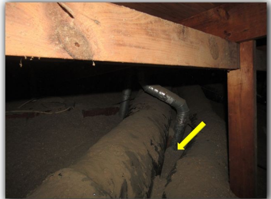
Appears flue for hall bathroom water heater contacts insulation
