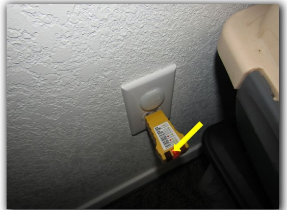
All of the two pong outlets and most of the three pong outlets are on a two wire system with no ground
