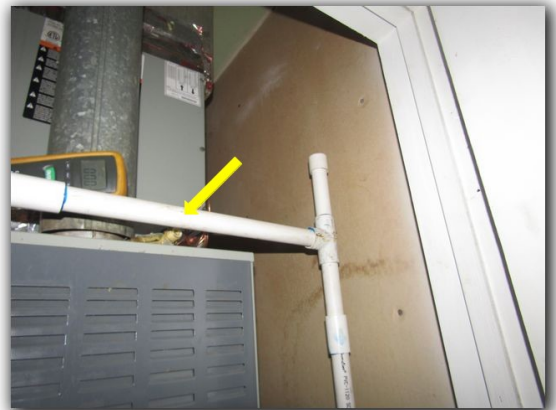
Recommend traps on A/C drain lines
