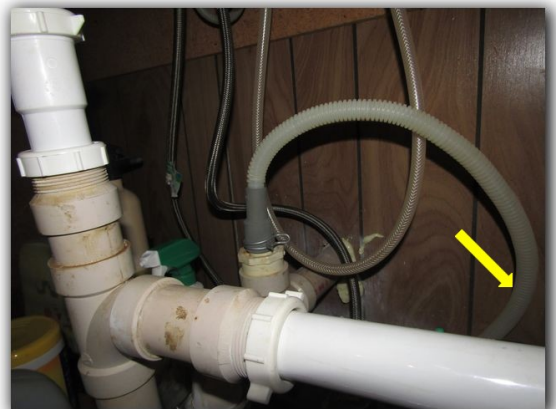
Dishwasher Drain line should be elevated or an anti-syphon device be installed to prevent backups from contaminating the dishwasher
