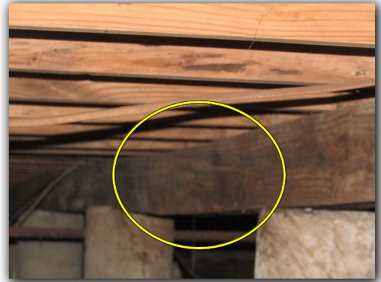
Possible damaged and warped beams observed in crawlspace
