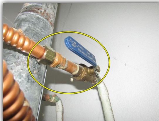
Possible corrosion observed at cold water supply valve for kitchen water heater
