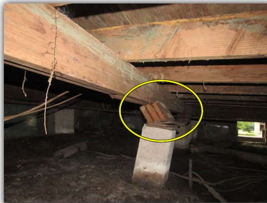
Multiple tilted piers observed in crawlspace
