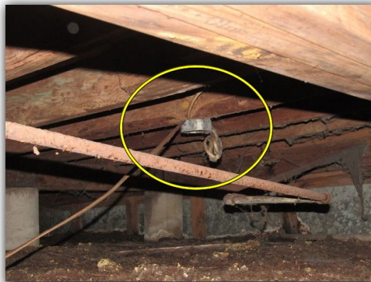
Recommend wiring in attic and crawlspace be in junction boxes
