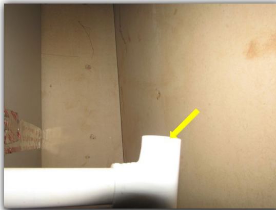
Recommend traps on A/C drain lines
