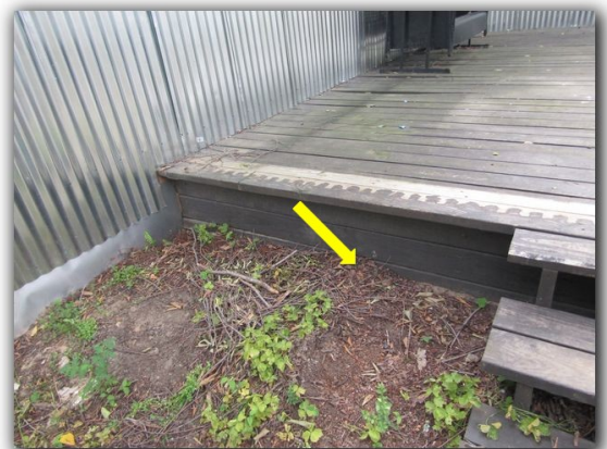
Wood to soil contact observed at back deck, front porch and side porch
