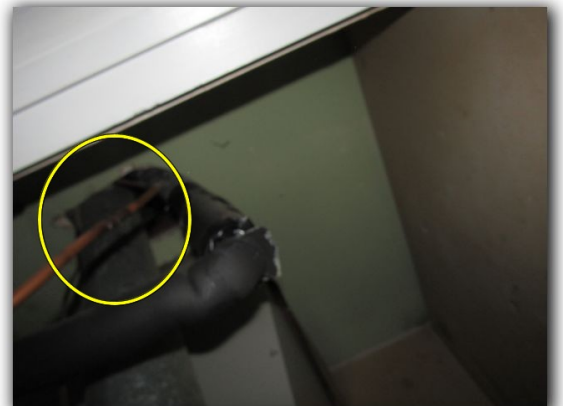
Flues for furnaces contact insulation
