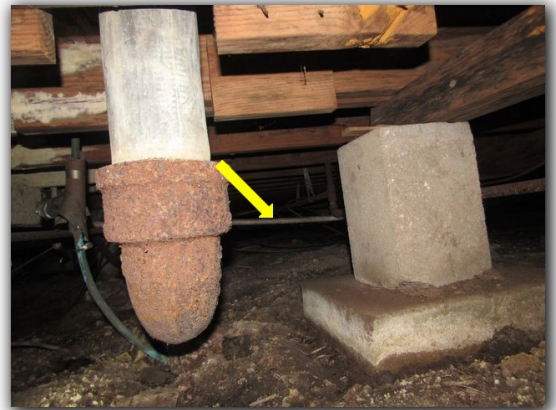
Appears A/C drain line is tilts back towards A/C unit in crawlspace and not towards termination
