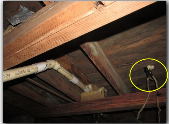
Recommend wiring in attic and crawlspace be in junction boxes
