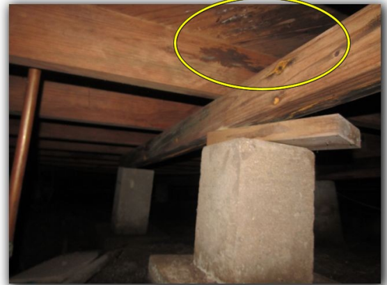
Possible damaged floor joist and signs of past leaks observed in crawlspace
