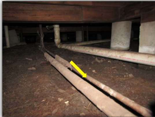
Supply lines in crawlspace should be covered with insulation
