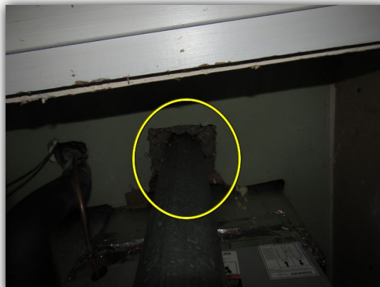
Flues for furnaces contact insulation
