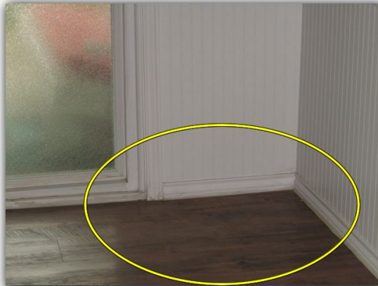
Slopes and dips observed at multiple locations in floor
