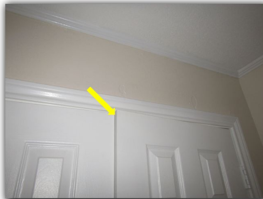
Multiple doors do not close completely or do not latch shut
