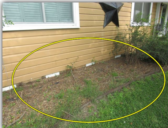
Appears grading on east side of home is flat or slopes toward home. Appears water may pool near home and enter crawlspace
