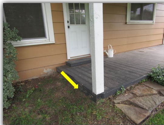
Wood to soil contact observed at back deck, front porch and side porch
