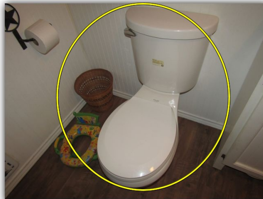
Hall bathroom toilet loose at base
