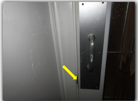
Multiple doors do not close completely or do not latch shut
