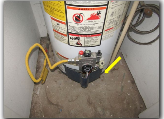
No drain pan underneath water heaters
