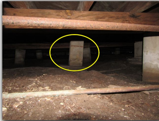
Multiple tilted piers observed in crawlspace
