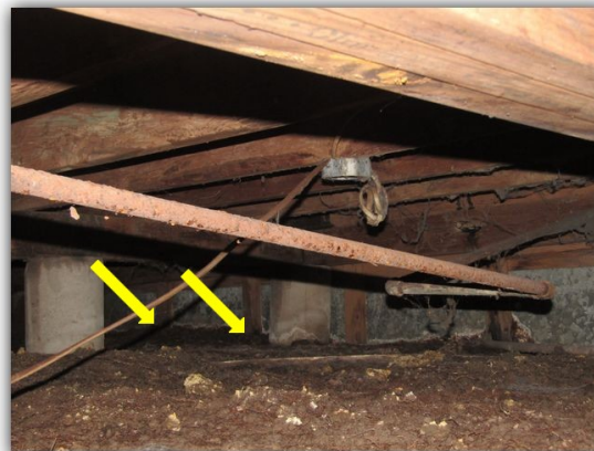
Wood to soil contact observed in crawlspace
