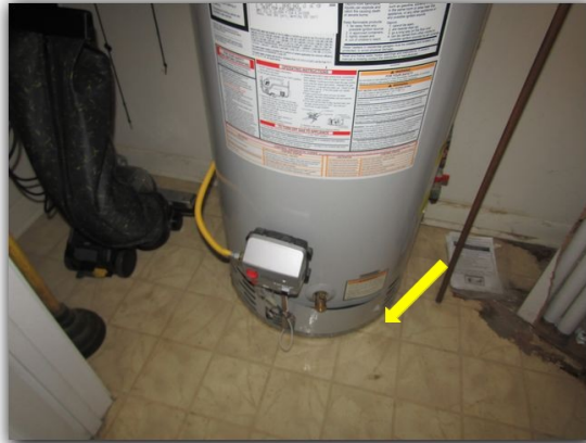
No drain pan underneath water heaters
