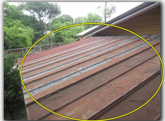
Rust observed on roofs for back and side porches
