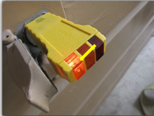
Carport receptacle is on an open neutral
