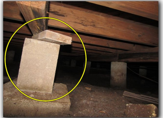
Multiple tilted piers observed in crawlspace
