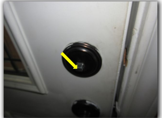
Appears entry door at carport is missing hardware
