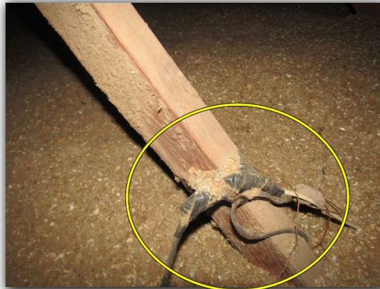
Recommend wiring in attic and crawlspace be in junction boxes
