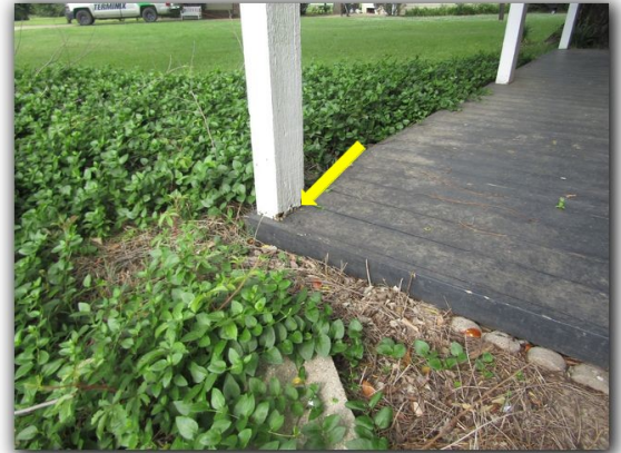
Possible damaged wood observed at side porch
