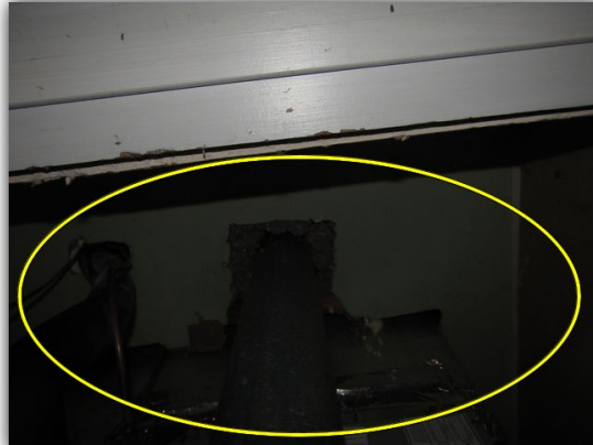
Due to gas furnaces. A/C closets should be vented
