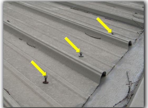
Appears multiple screws are loose on roof
