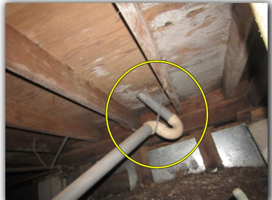
Old drain pipes observed in crawlspace
