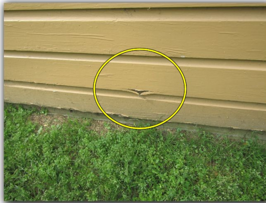
Possible damaged wood siding observed
