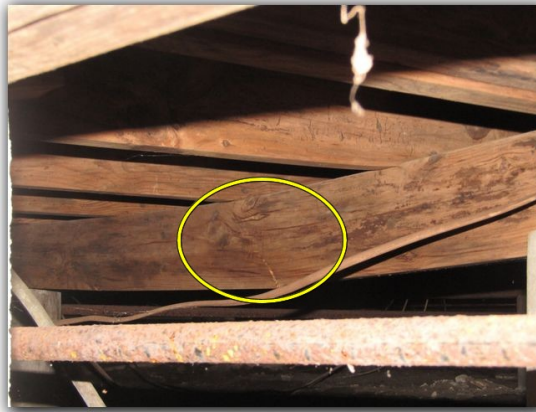
Possible damaged and warped beams observed in crawlspace
