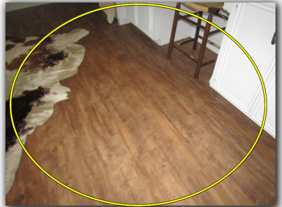
Evidence of past leaks observed on ceiling in kitchen hot water closet
