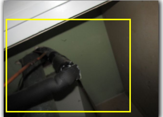
Due to gas furnaces. A/C closets should be vented
