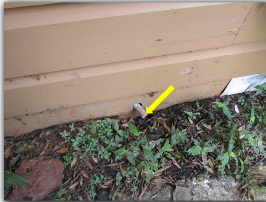
A/C drain line terminates to exterior.
