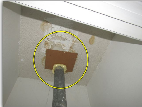
Recommend heat shield at kitchen water heater
