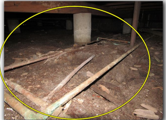
Supply lines in crawlspace should be covered with insulation
