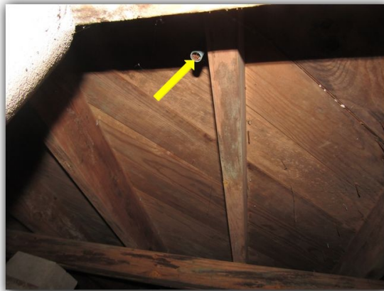
Drain line for hall bathroom water heater temperature pressure relief valve terminates in crawlspace.
