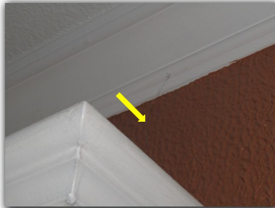
Cracks in interior walls observed
