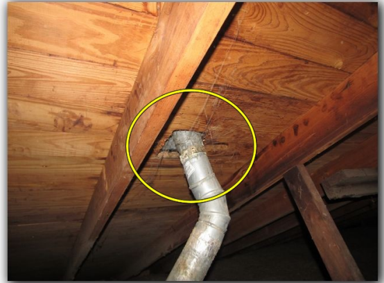
Evidence of past leaks observed in attic
