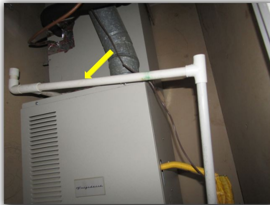
Recommend traps on A/C drain lines
