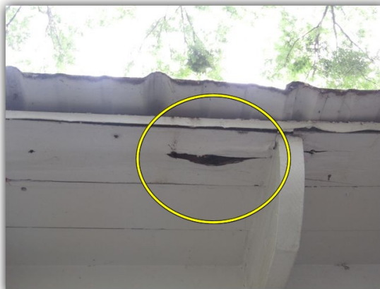
Possible damaged wood observed at eaves
