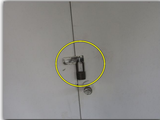
Unable to inspect carport storage closet. Closet was locked at time of inspection
