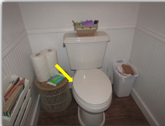
Supply valve for master toilet was turned off at time of inspection.
