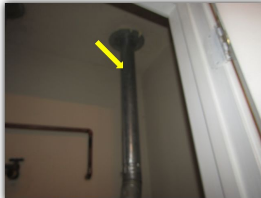
Appears to be a flue no longer in use in hall bathroom water heater closet
