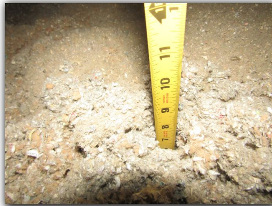
Average Depth of Insulation is 8 Inches
