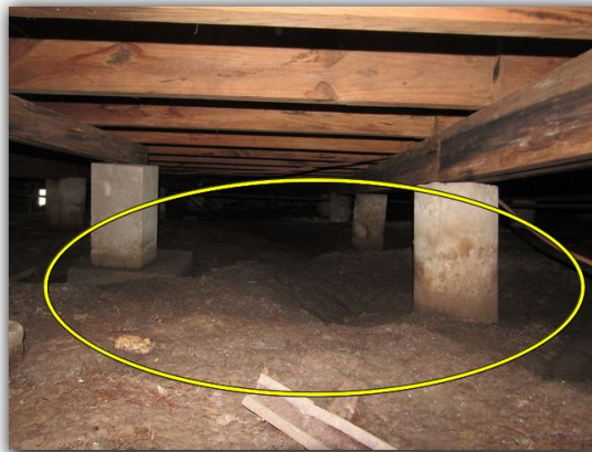
Possible poor drainage in crawlspace. Appears water may enter crawlspace and pool in multiple locations in crawlspace.
