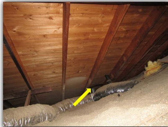
Average Depth of Insulation is 8 Inches
