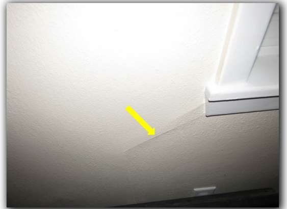
Cracks in interior walls observed
