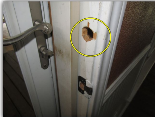
Appears entry door at carport is missing hardware
