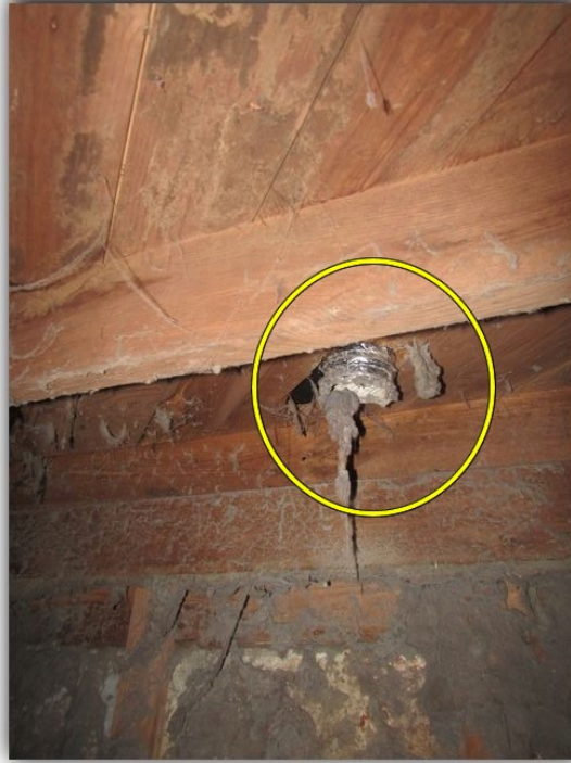
Dryer vent terminates in crawlspace
