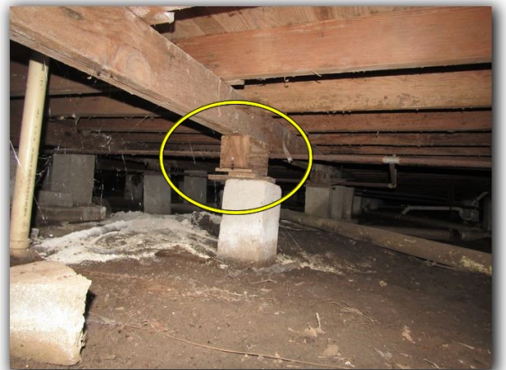
Multiple tilted piers observed in crawlspace
