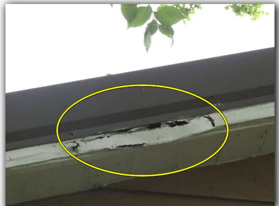
Possible damaged wood observed at eaves
