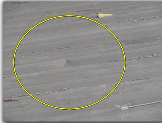
Multiple dents in roof observed
