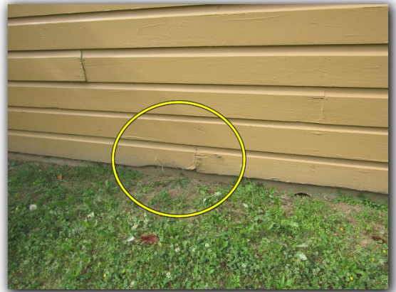
Possible damaged wood siding observed
