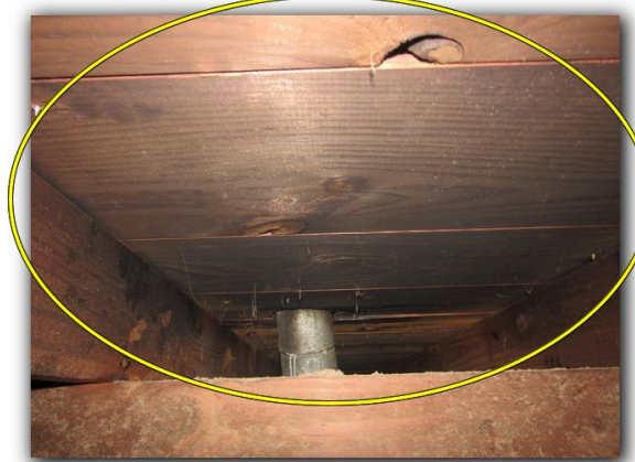
Possible soot observed in attic at furnace flue
