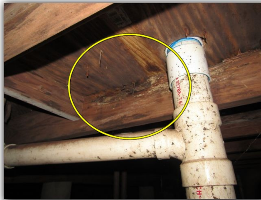
Possible damaged floor joist and signs of past leaks observed in crawlspace
