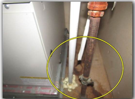
Recommend traps on A/C drain lines
