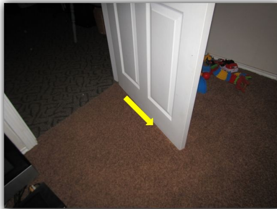
Appears door to office rubs against carpet and floor
