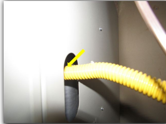
Flex connector enters left furnace
