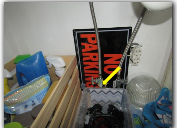
Possible corrosion observed on hot water supply valve under master bath sink
