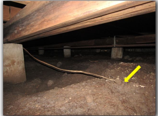
Recommend wiring in crawlspace not be on the ground
