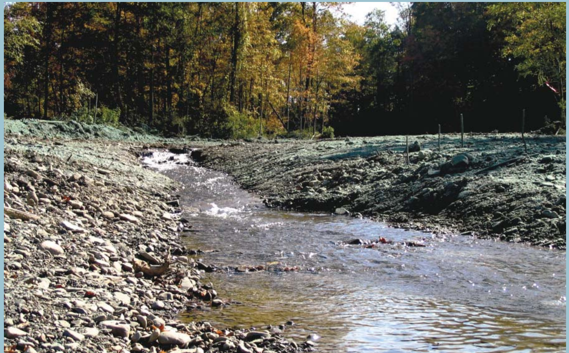
Six Mile Creek, streambank stabilization
