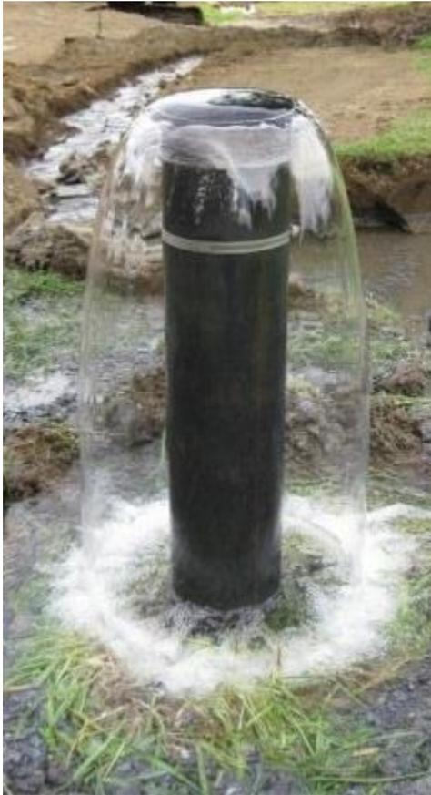
However, all this can be avoided by controlling the flowing well. This might be accomplished simply by adding a few feet of well casing to the top of the well or by following other standard well drilling industry practices to stop the flow while maintaining its use. Owners of flowing wells should enlist the aid of a [NYSDEC registered well driller](#) to ensure the proper operation of groundwater wells. [NYSDEC regulations](#) address the damage caused by uncontrolled flowing wells, including:
