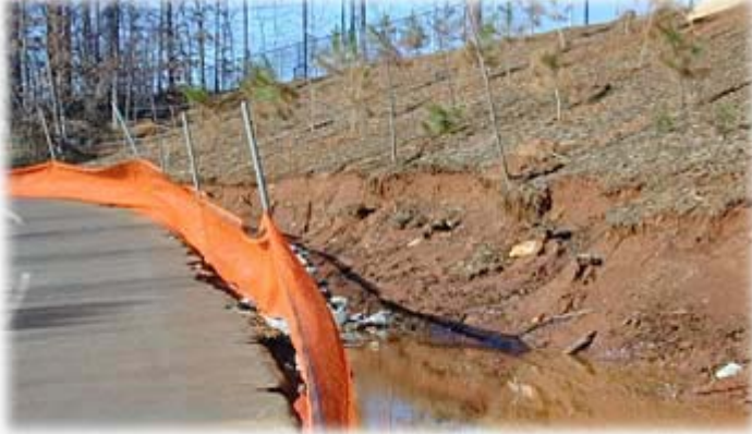
Erosion caused by surface runoff
