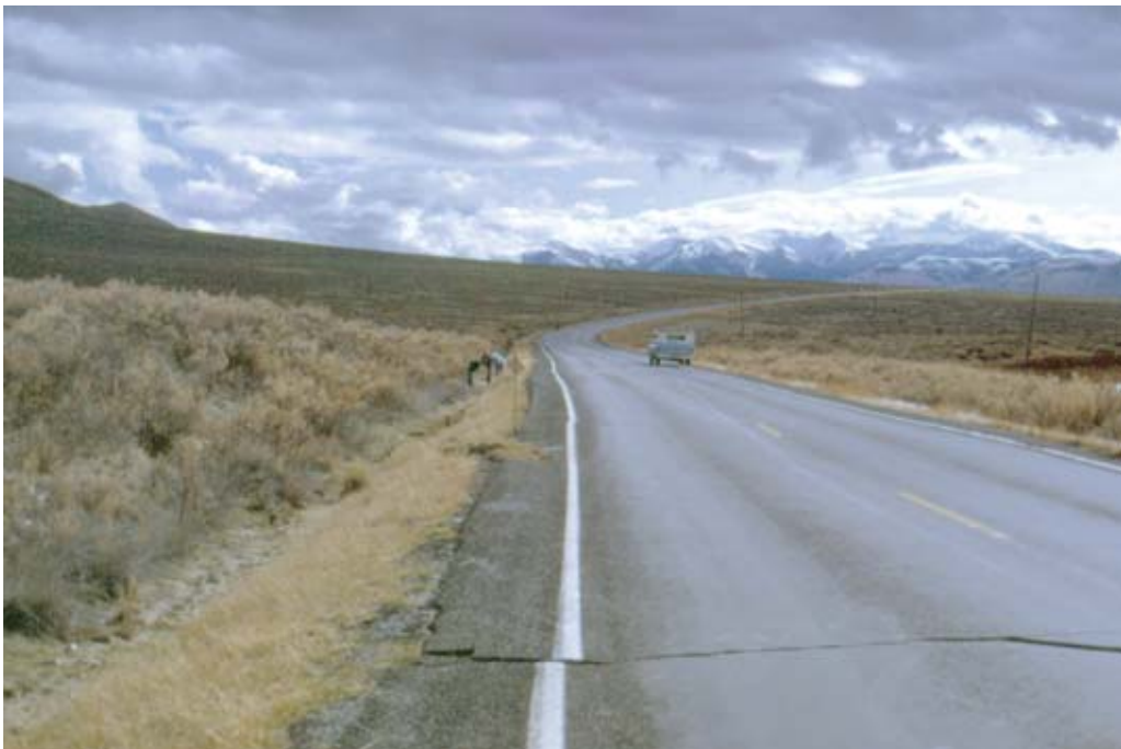
Highway offset by an earthquake fault in east-central Idaho. (Photo by Karl Hipple, USDA, NRCS.)
