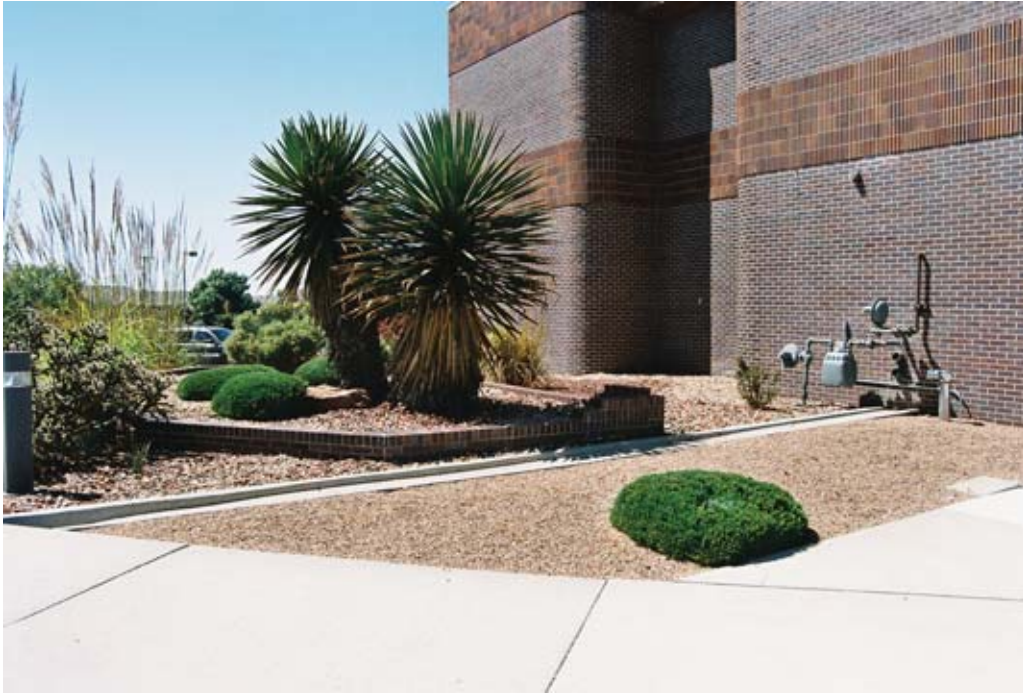
Low water-use landscaping and drainage away from buildings help to prevent soil collapse. (NRCS photo.)
