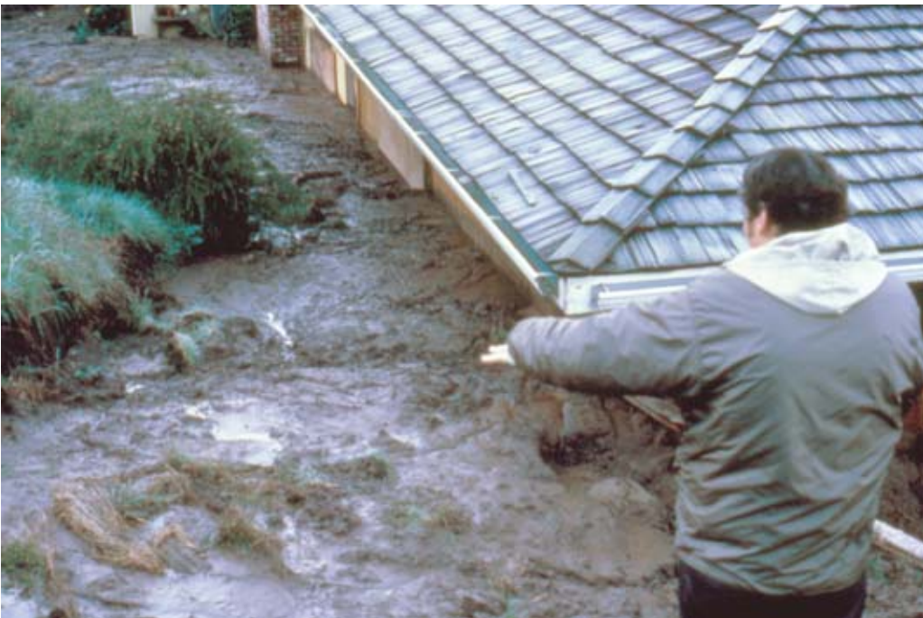
Soil debris from a landslide. (NRCS photo.)
