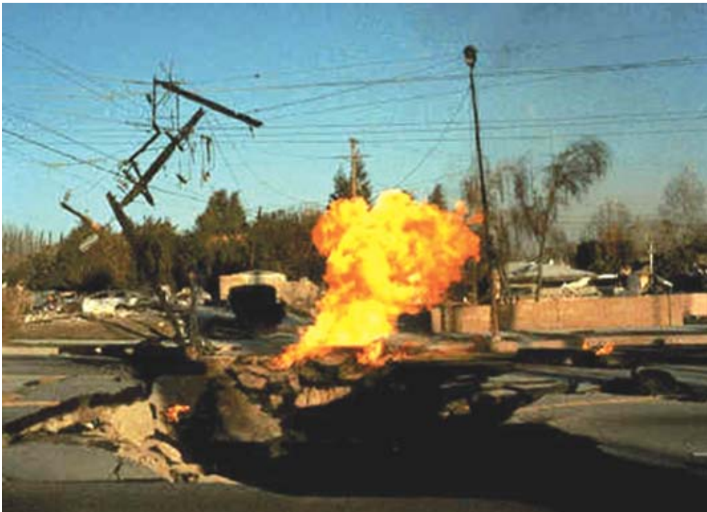
California earthquake of 1994. (USGS photo.)
