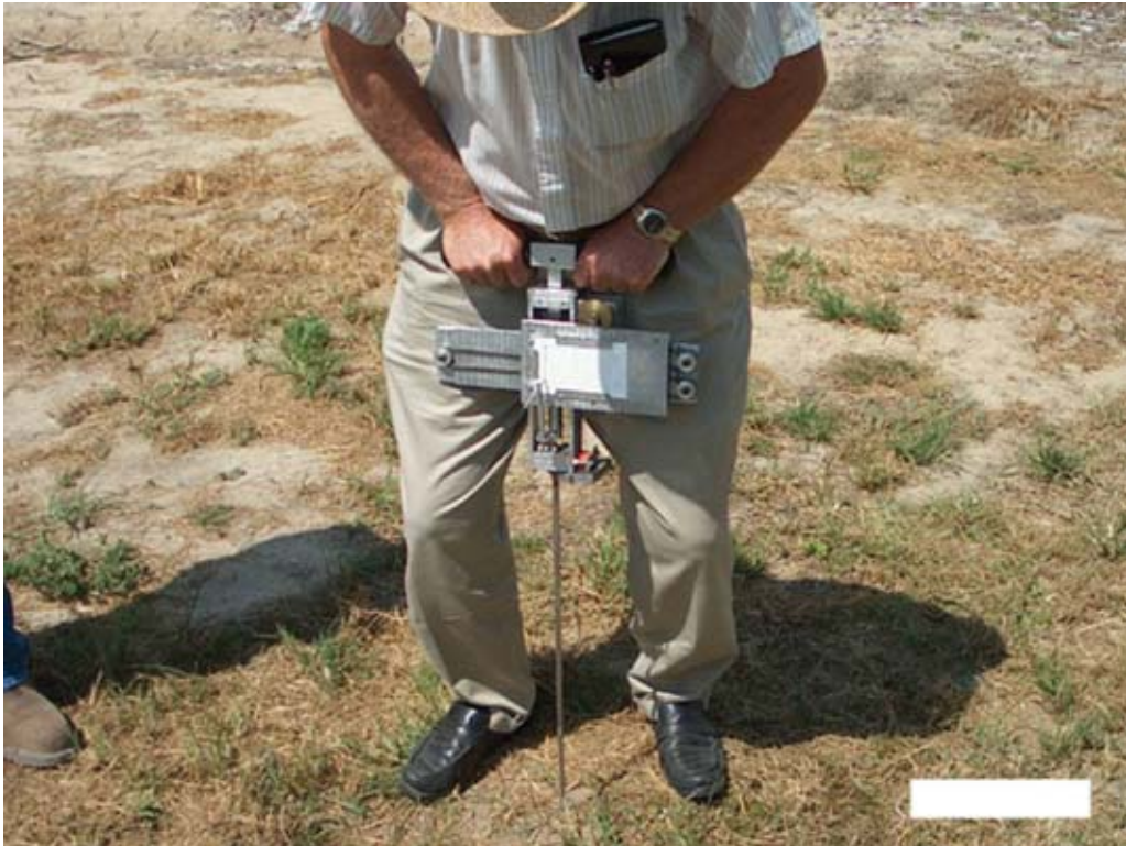
Using a penetrometer to check compaction.
