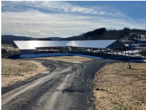
Photo 3: The new covered barnyard and waste storage facility. The left side of the structure is the covered barnyard and the right side is the waste storage facility
