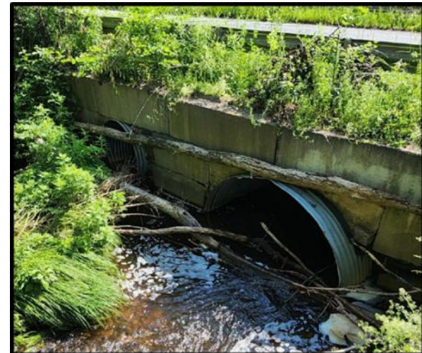
Figure 2 View of Gun House Hill Road double culvert inlets. Note the woody debris caught by the undersized culverts.
