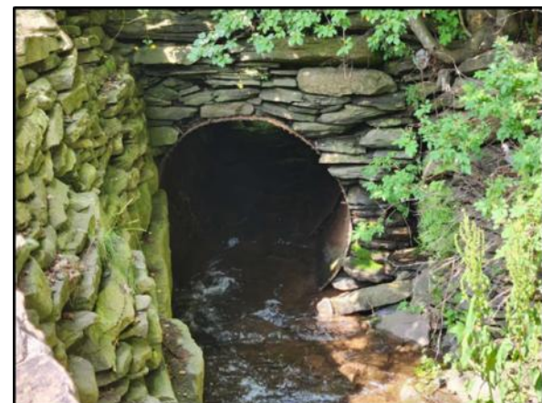
Figure 3 View of Maple Avenue culvert inlet with the constricted opening. The Grant Brook stream channel narrows down to the metal boiler plate culvert inlet.
