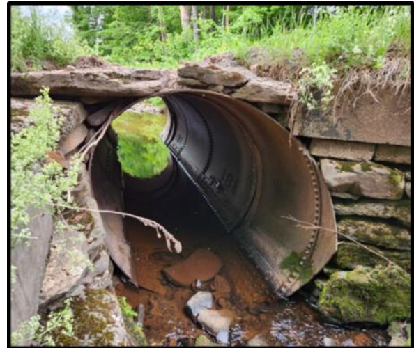
Figure 1 View of Reed Road culvert inlet. Note the boiler plate structure is misshapen and the bottom is rusted through.
