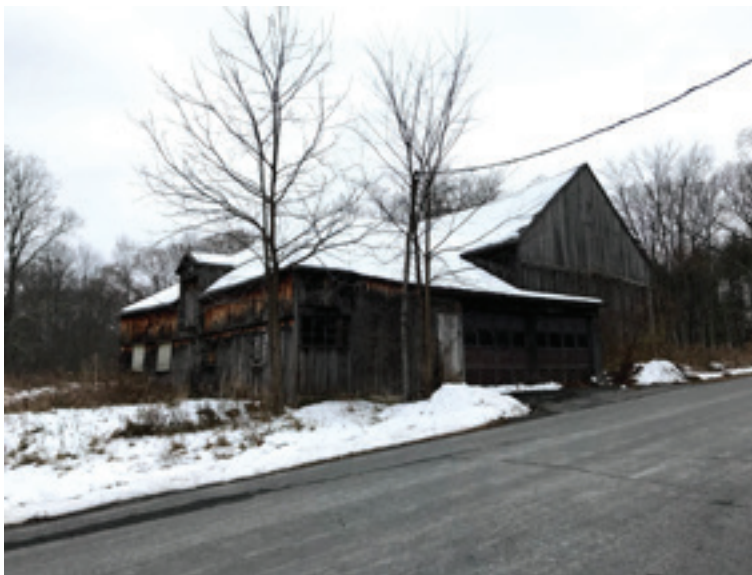
The barn at Bluebird Farm before renovation.
