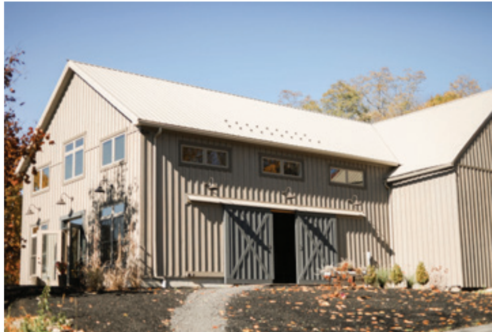
The renovated barn at Bluebird Farm.
