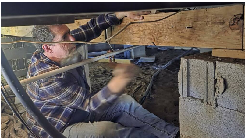
Pastor Troy working underneath the multipurpose building in Carthage.
