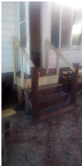
Steps installed at the multipurpose building at Shiloh Tabernacle in Carthage, NC
