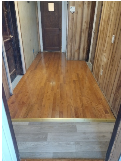
After new flooring install in foyer
