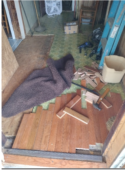
Installing new flooring at Fellowship Hall in Carthage
