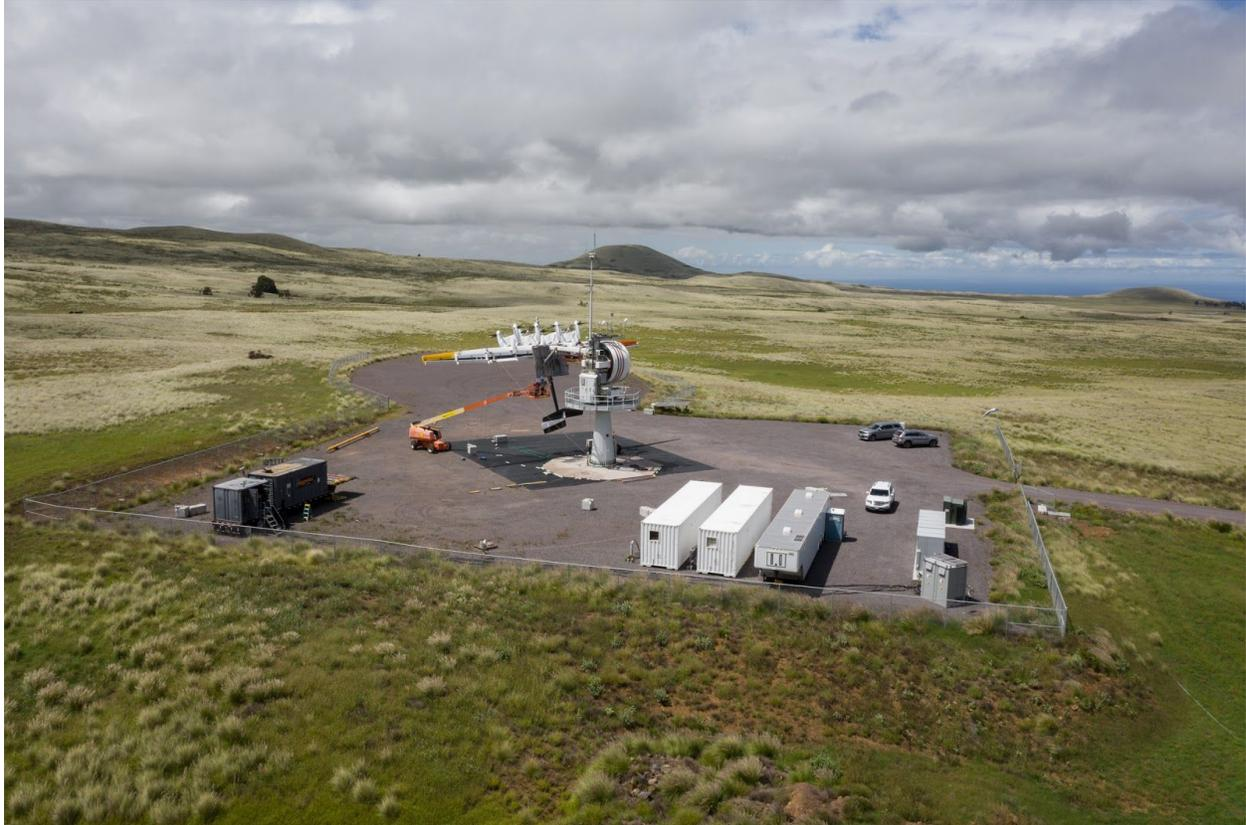
**Figure 8: Hawaii Test Site in 2019. This drone photograph shows the 5 m tower and kite SN4 sitting on the perch of GS02. In the foreground are the ground power inverters and the switchgear to the HELCO electrical grid.**
