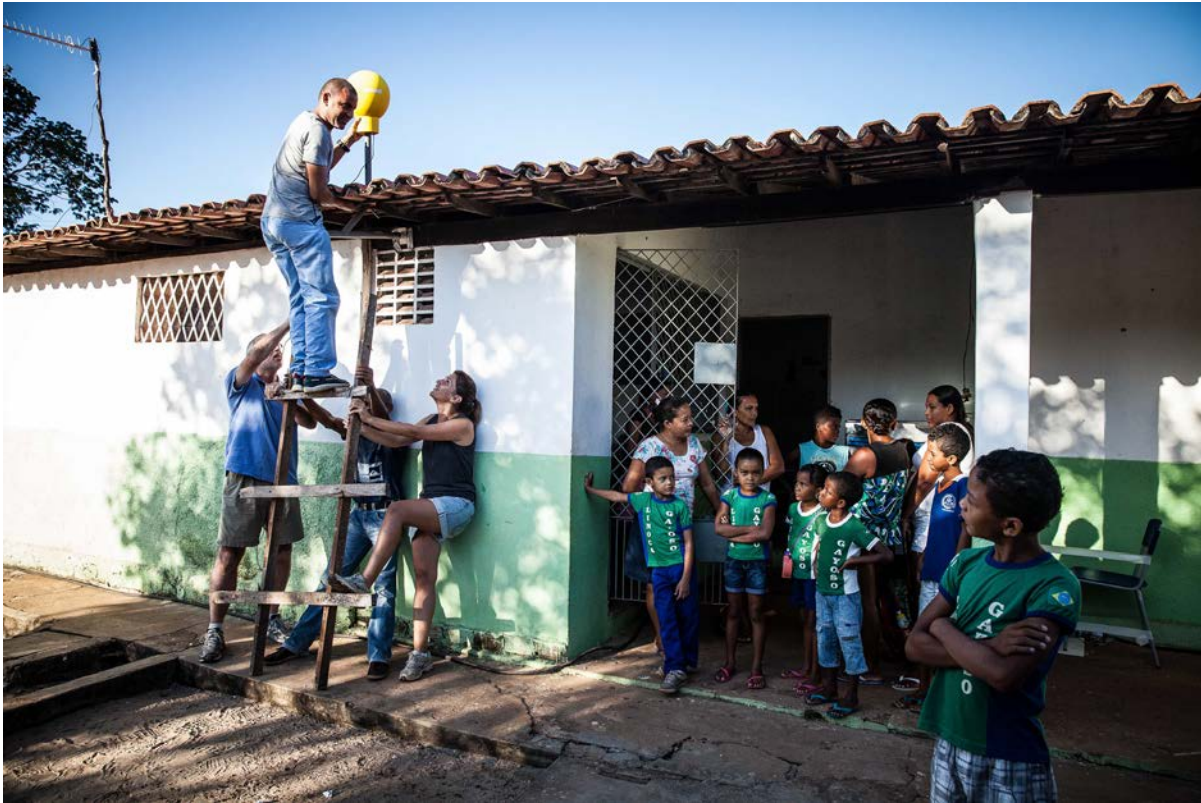
Figure 4-1 Early Loon fixed wireless service. Installing terminals on roof of school in Agua Fria, Brazil.
