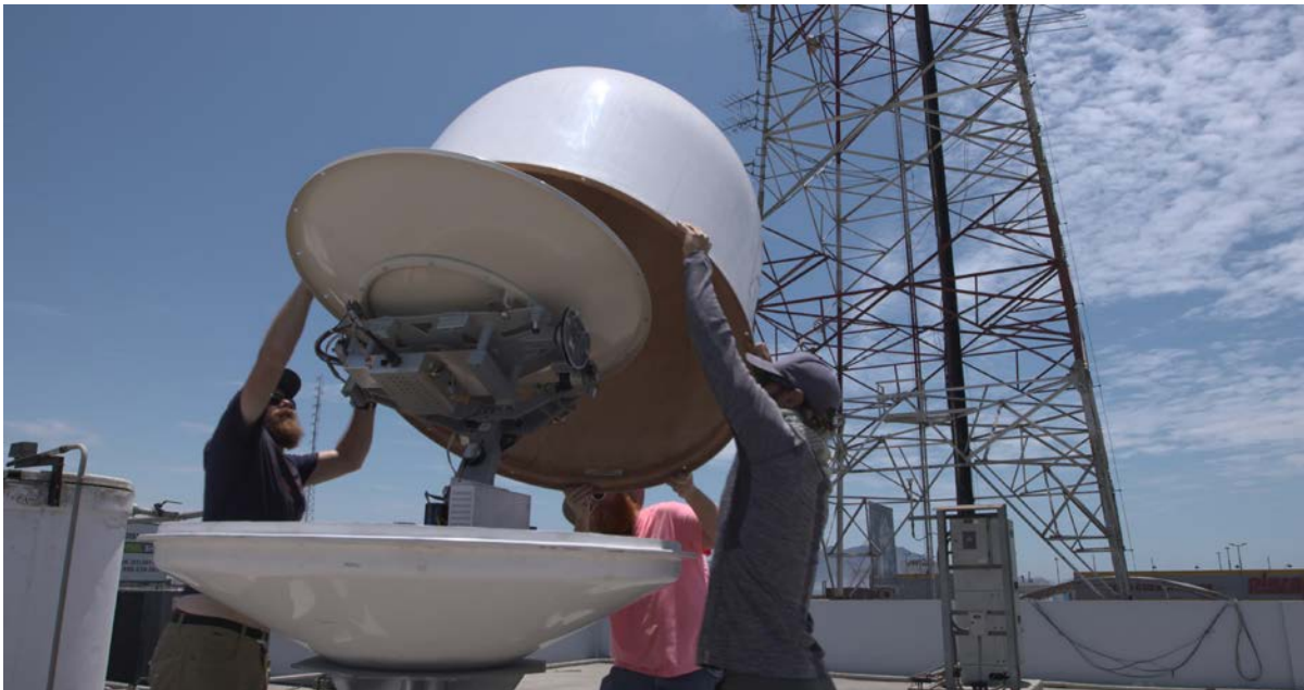
Figure 4-37 Installation of radome on Loon Ground station.
