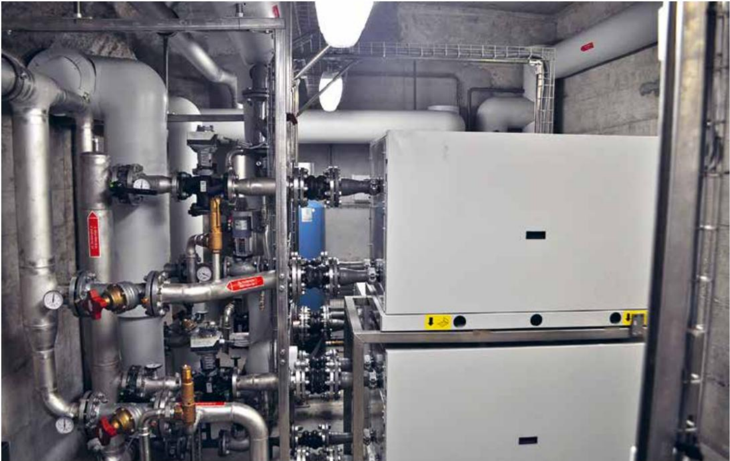
Heat pumps and heating pipes
