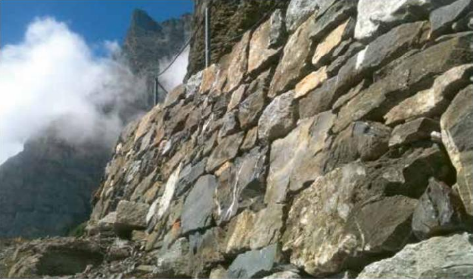
Example of a dry stone wall, expertly stacked by the specialist company Schteimüürini.
