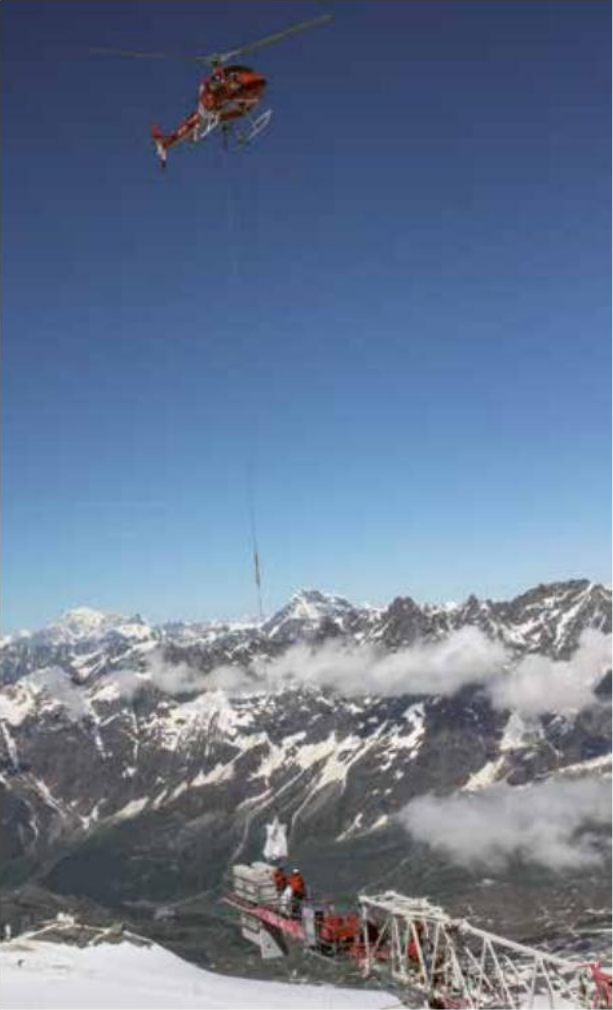
Crane assembly: Air Zermatt pitched in. To assemble the crane erect, the parts had to be transported by helicopter become.
