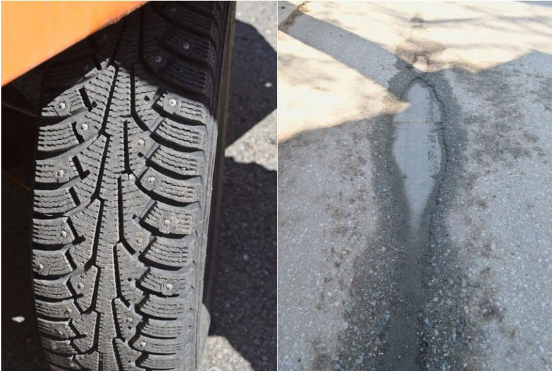
Studded tires cause significant wear on the road surface.
