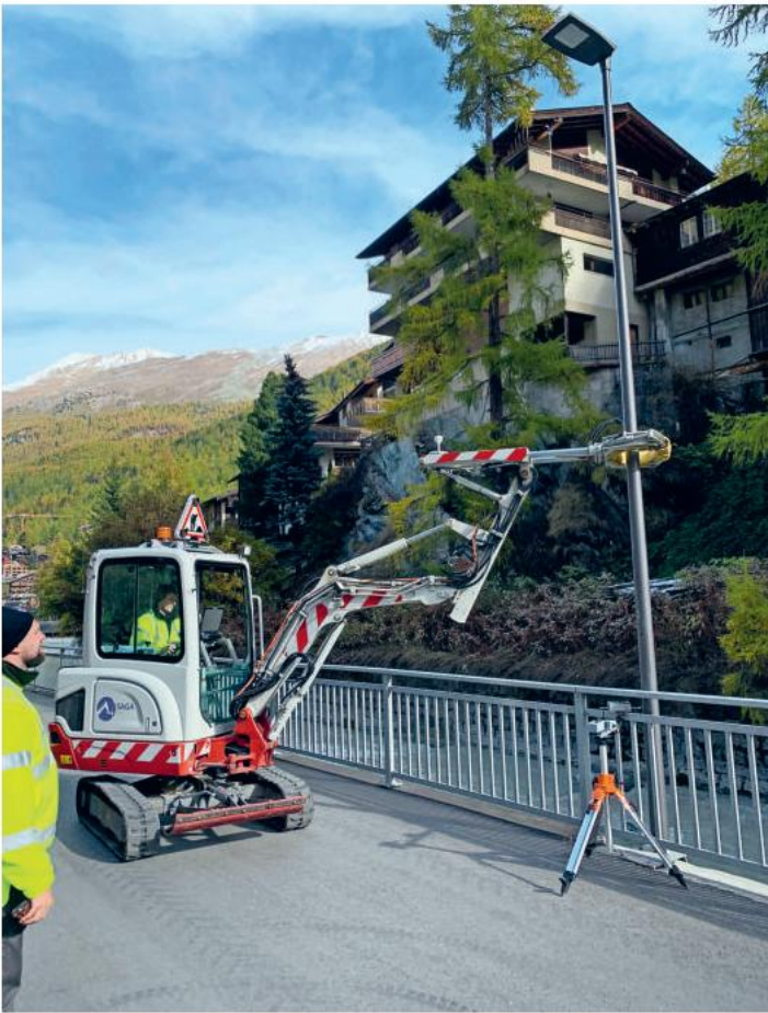
Candelabras are tested for stability.
