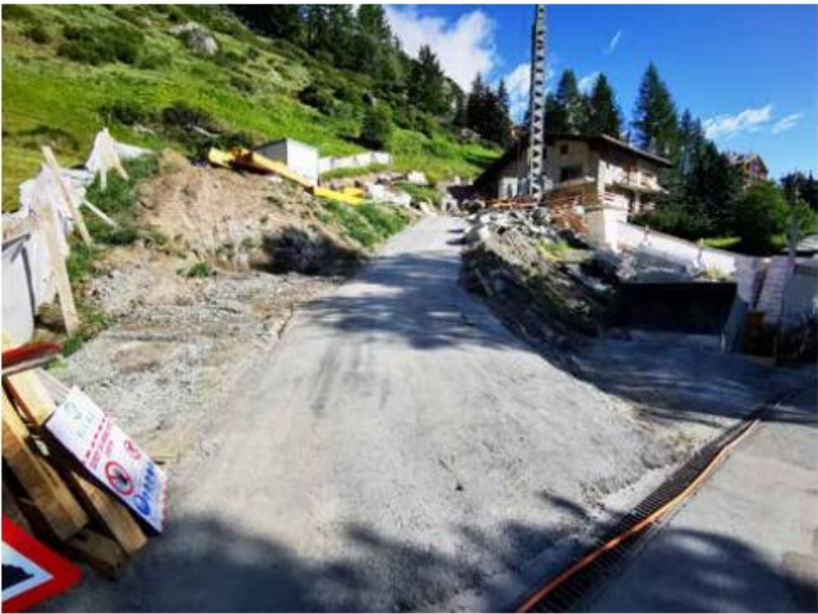
Example of a compacted construction site access road Photo: EWG
