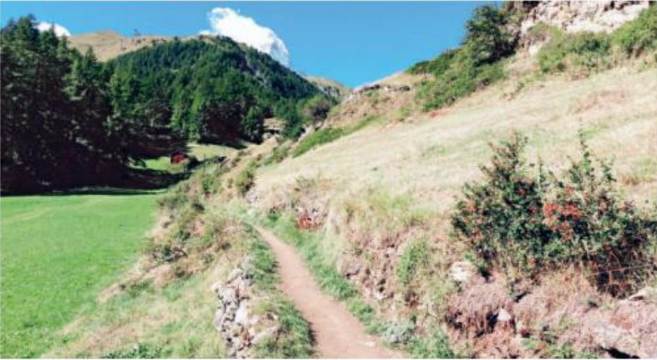
Situation in autumn 2023: Due to their age, the dry stone walls are in poor condition, heavily overgrown and slowly decaying.
