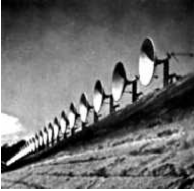
An early interferometric radio telescope at the University of Sydney, Australia ( N = 32 , \lambda = 21 cm, d = 7 m, 2 m diameter, 700 ft. east–west base line). (W.N. Christiansen)
